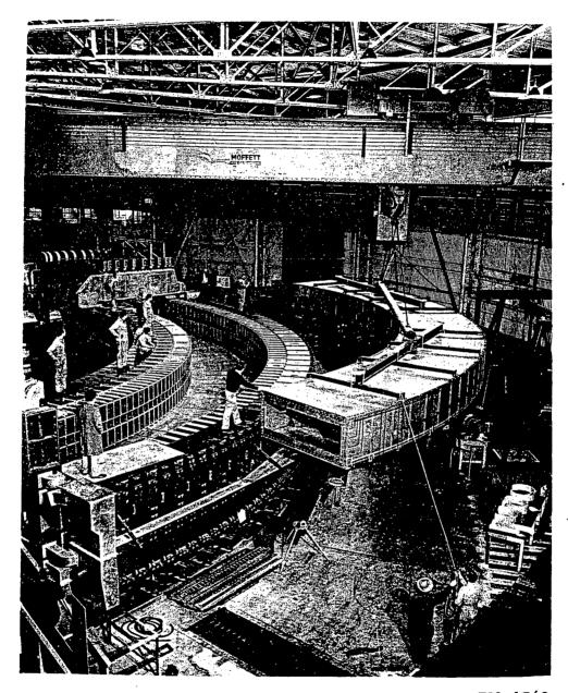
Fig. 4. Installing a vacuum tube. Note pump-out lines on sides of tank.
