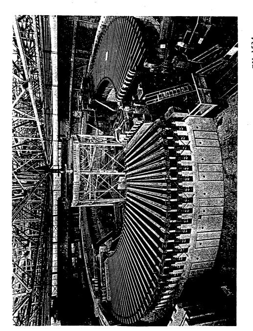
8. Over-all view of the Bevatron. The straight section in the foreground is used for injection, that at the far right for acceleration, and the one at the left for the induction Fig. 8. Over-all view of the Bevatron. electrodes.
