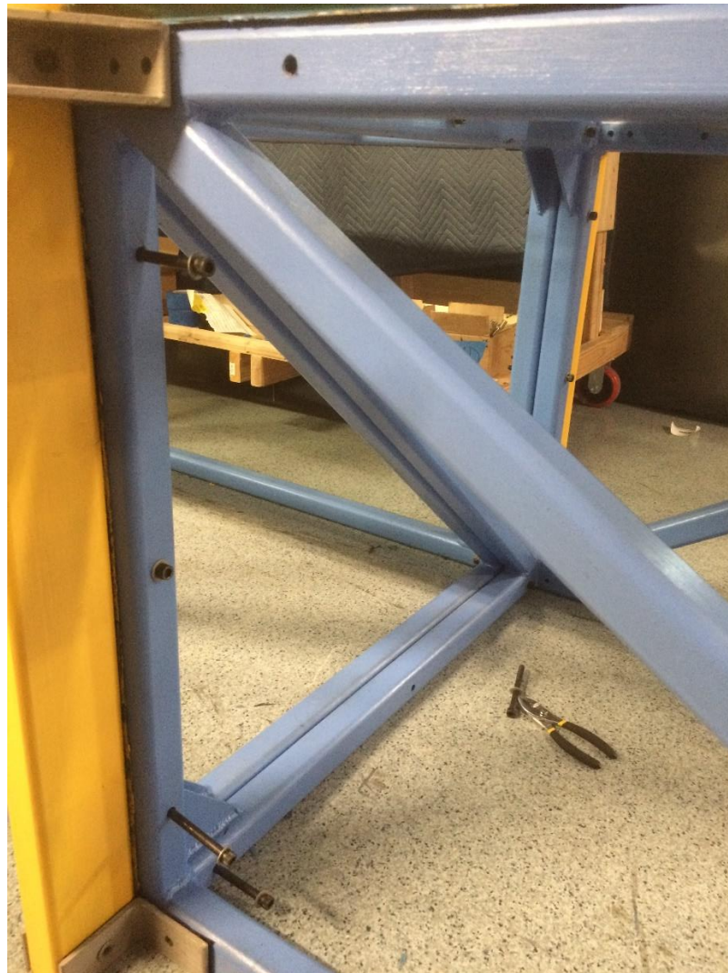
Figure 5.11: Bolt misalignment between second and third chassis module.
