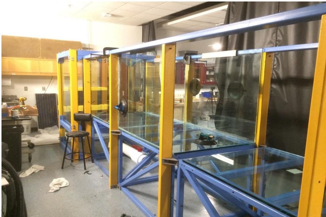
Figure 5.10: Second section completed.
