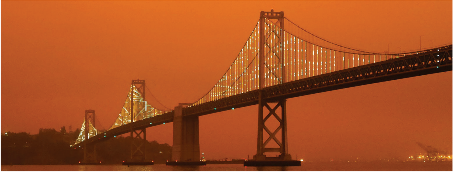
San Francisco Bay Bridge in 2020 when the sky turned orange during wildfires
