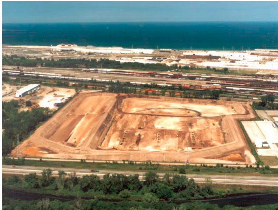
Figure 1.1 Aerial photo of confined disposal facility at Grand Calumet River in Gary after grading (Lee 2007).
