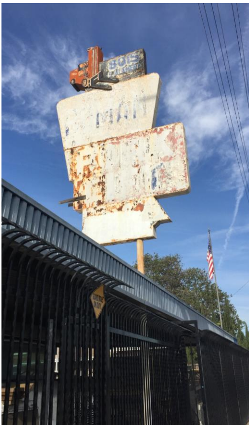
Above: An illegible sign makes it difficult to see what business is located on the premises. It makes it more difficult to raise complaints about potential problems with the site.
