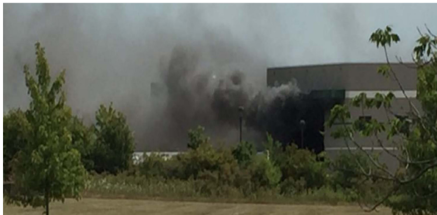
Figure 21. BESS Fire at S&C Electric Manufacturing Facility in Franklin, Wisconsin (WPI report photo)
