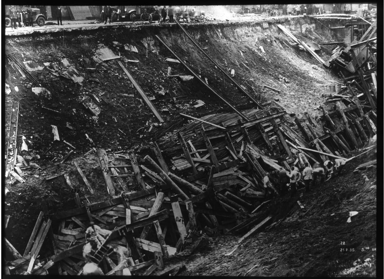
Fig. 32. Degebo. Photograph of a landslide in a railway cutting at an unspecified location. 21 Aug 1935. Diaarchiv Degebo.
