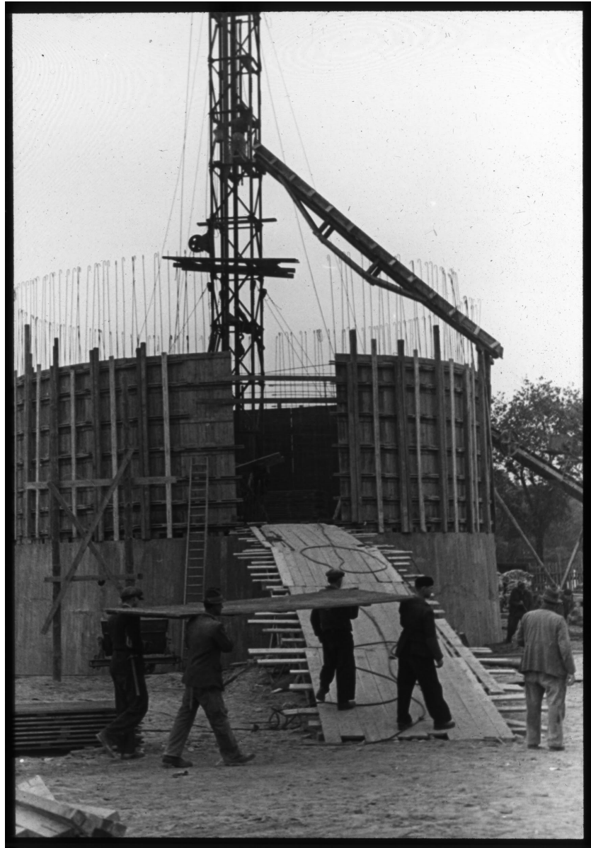
Fig. 80. Degebo. Forced laborers carrying parts of the cylinder's shell construction. 1941.
