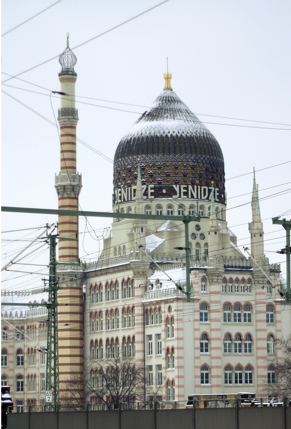
Illustration 3.01: Recent image of Yenidze cigarette factory. Today the building no longer serves its original purpose.
