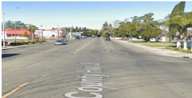
a) Franklin Blvd, before transforming to a complete street (currently) (Google map, 2020)
