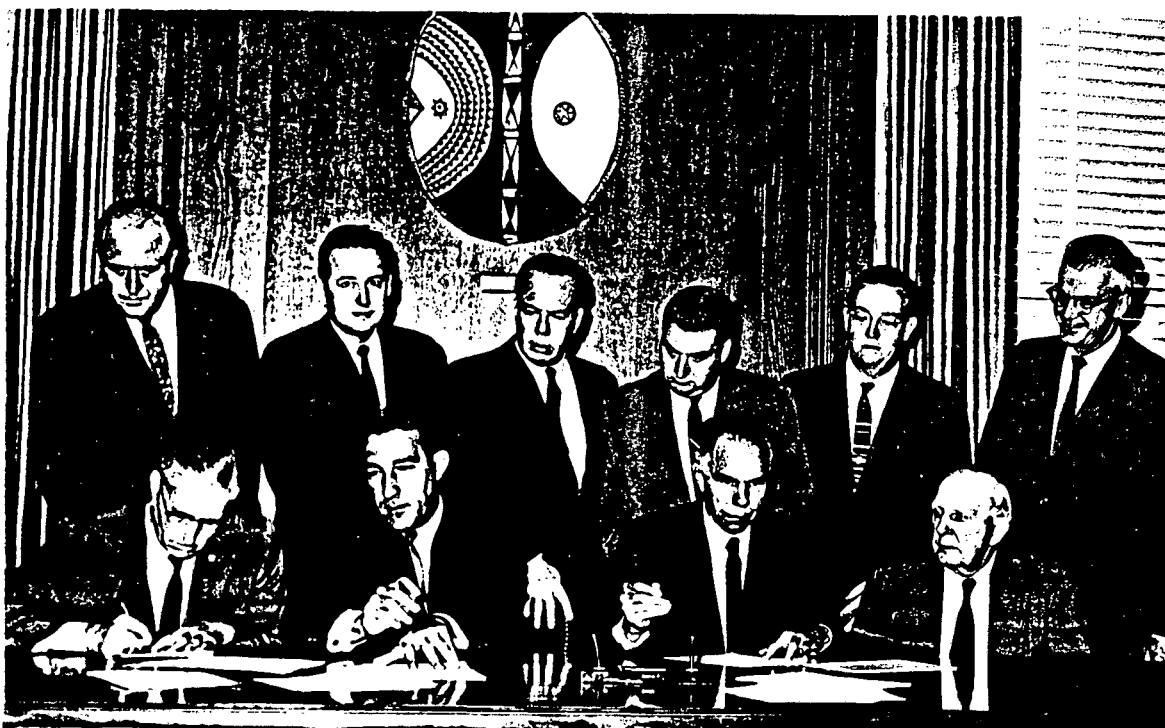
Contract signing for study of sea water conversion plant, August 18, 1964
