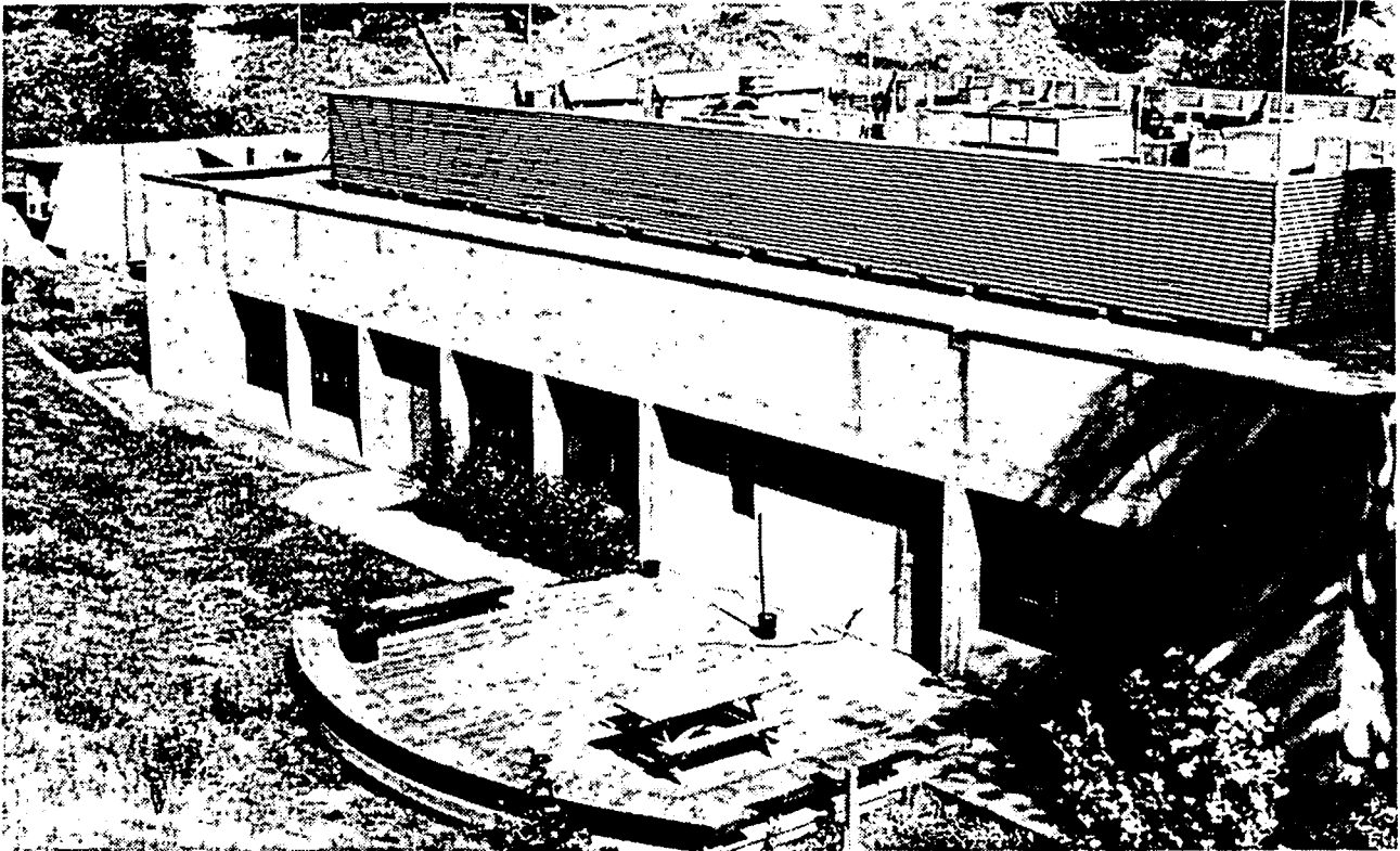
A. Uncluttered architecture and equipment screening are typical of Buildings 83 and 74.
