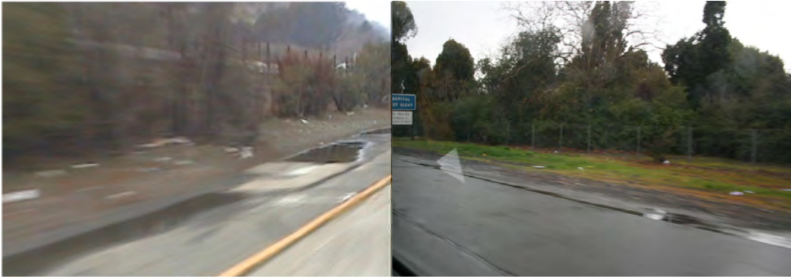
PHOTOGRAPH 1 Water Accumulation on Drivers' Left Shoulder and Heavy Vegetation at Study Site 1
