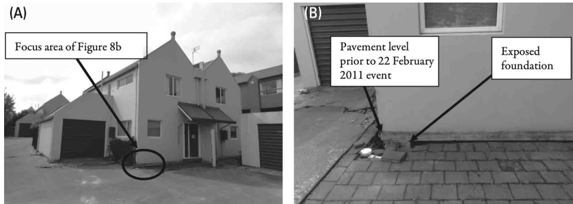
Figure 3.20: Duplex housing complex: A) looking north at the center building, and B) close-up of ground settlement next to the center building (16 March 2011; S43.52399 E172.64417) [15].
