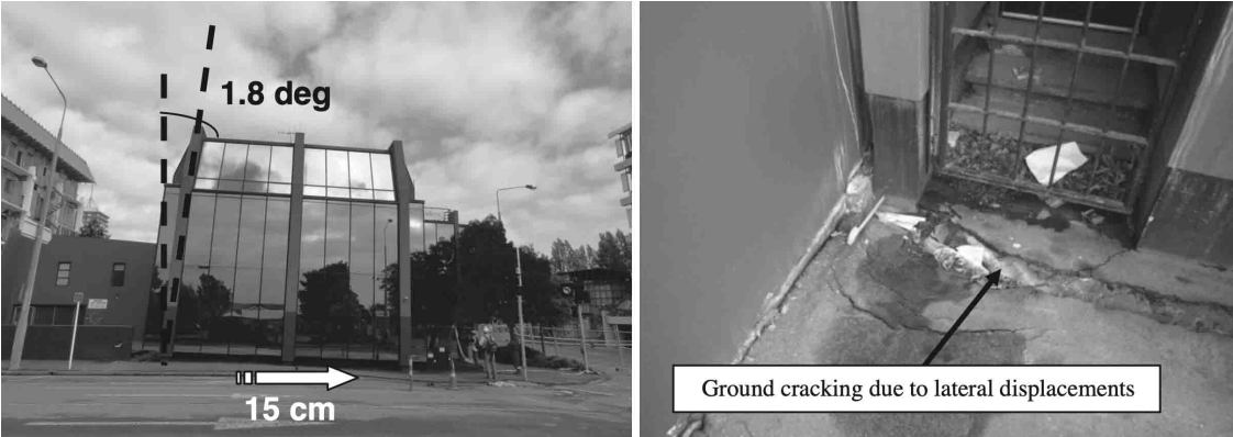
Figure 3.22: Liquefaction-induced differential settlement and sliding of building in the CBD (24 March 2011; S43.52878 E172.64252) [15].
