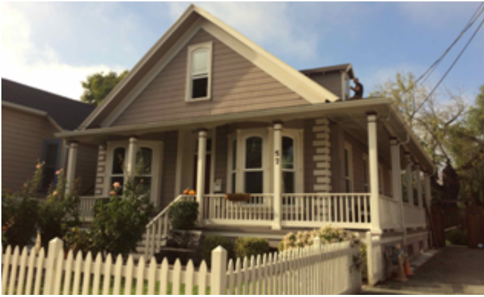
New windows being installed through out the whole house.
