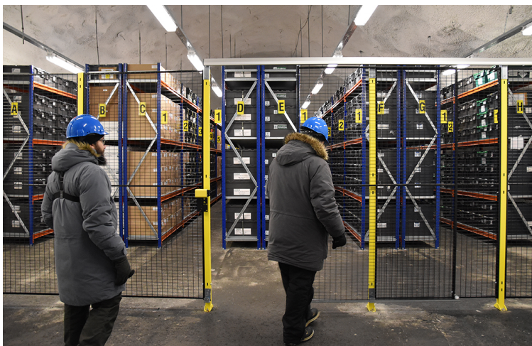
Figure 7. One of three refrigerated storage rooms for seeds collected from various agricultural institutes. The architecture is utilitarian: fluorescent lights, bare concrete walls and floor, a metal gate, and metal shelves that hold boxes of uniform, stackable sizes from multiple institutes.
