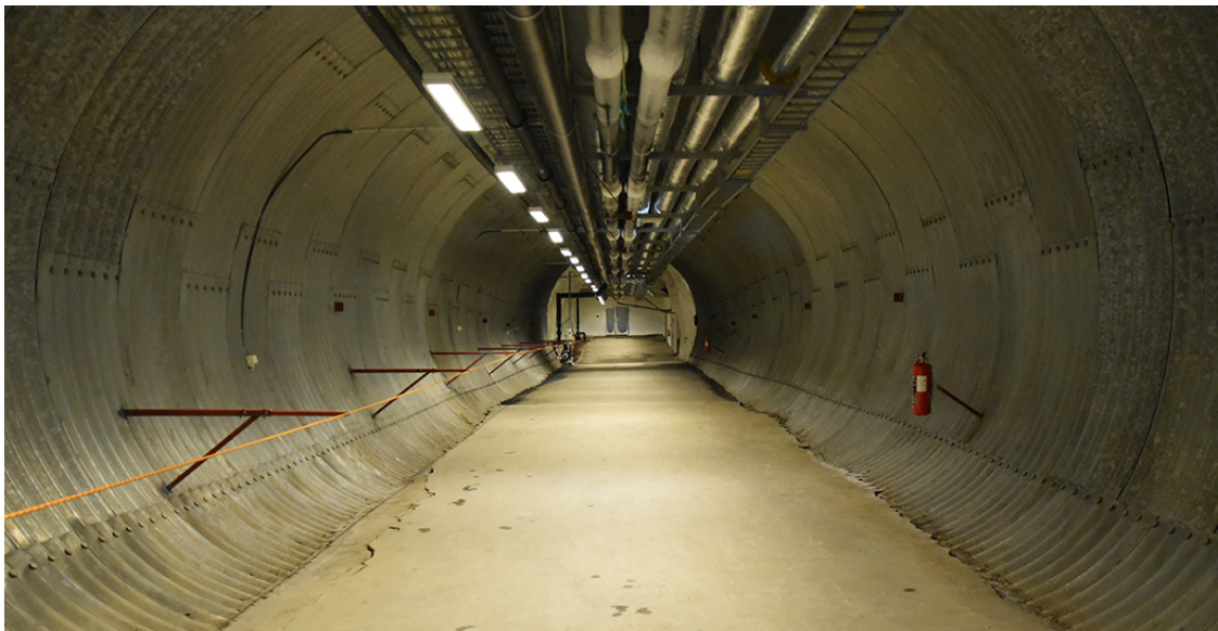
Figure 6. A hundred-meter tunnel leads to the entrance to three storage rooms at the vault. Its length is designed to protect the vault from outside attack (Gan, 2015).
