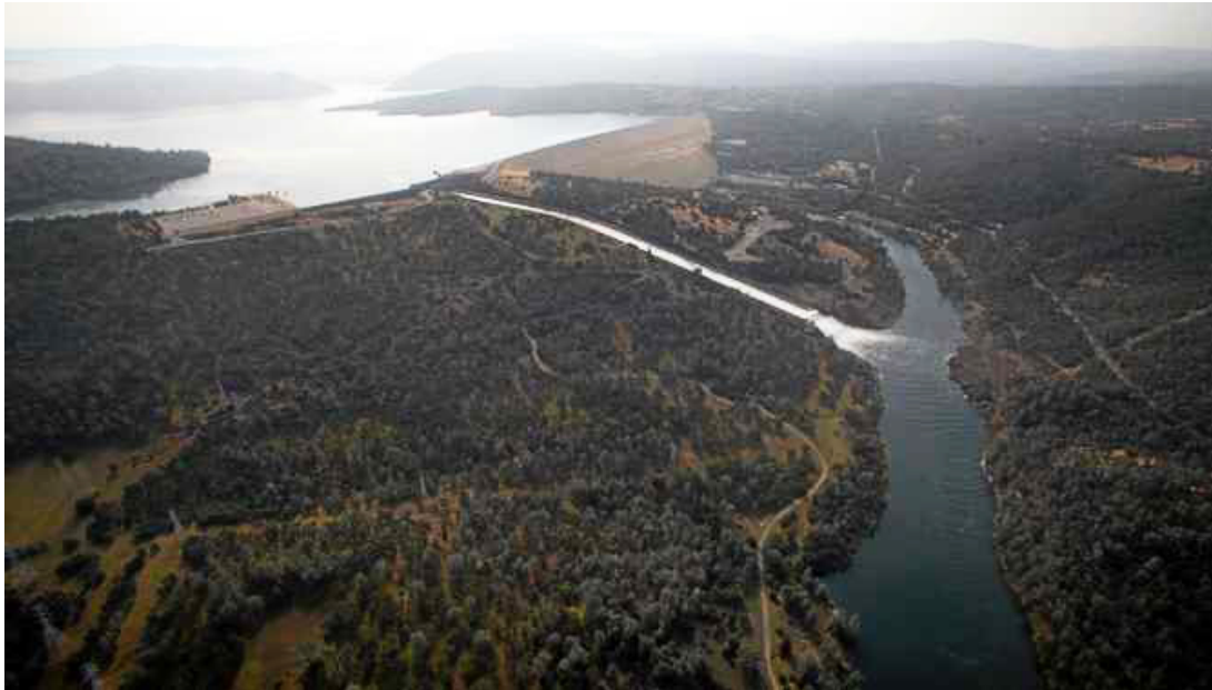
Figure 23. An aerial photograph of Oroville Dam, the tallest earthen dam in the U.S. and located east of the Sacramento valley. Snowmelt from the Sierra Nevadas and rainfall drain into a manmade reservoir, Lake Oroville (left). Water is released via a spillway (center) into the Feather River (right), a main tributary of the Sacramento River. The dam has significantly reduced the river's annual discharge, splitting it between agriculture in Northern California and hydroelectricity for Central and Southern California, and endangering the cycles of ecological niche constructors like beavers and steelhead salmon (Jason Halley, Chico-Enterprise Record, 2011).
