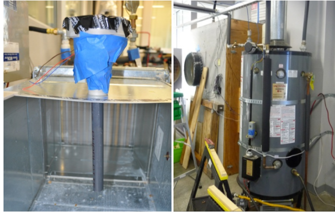
FIGURE 6 - DEVICE TO MEASURE DRY BULB TEMPERATURE AFTER THE SPRAY (LEFT) AND WATER HEATER (RIGHT)
