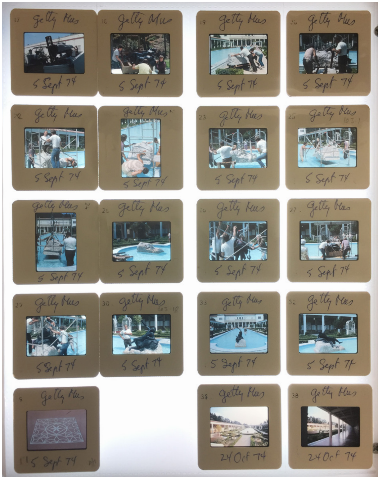
Figure 10. Slide sheet of installation of pool statue taken by Norman Neuerburg, 5 September 1974, Box 16, Norman Neuerburg papers regarding Getty Villa design and construction, 1966-1987, bulk 1970- 1975, Getty Research Institute, Los Angeles, California.
