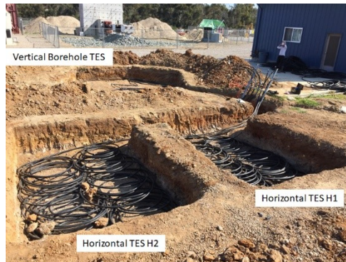
Figure 3. Picture of the UCSD thermal energy storage (TES) systems before backfilling
