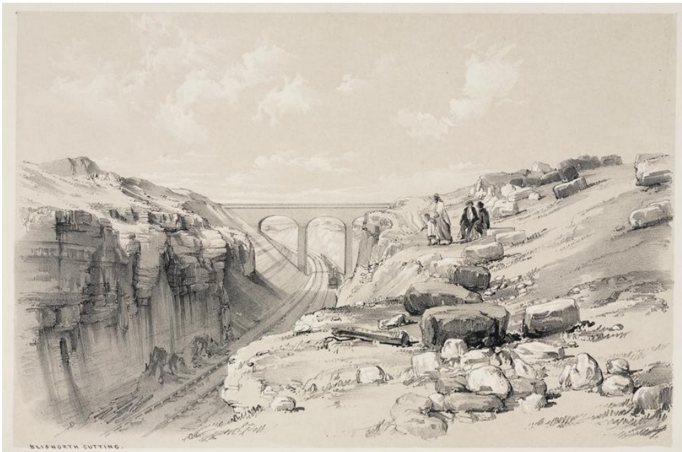
John Cooke Bourne, Blisworth Cutting – A View from Above , Plate XXVI from Drawings of the London and Birmingham Railway (London: JC Bourne, Ackermann & Co, 1839)
