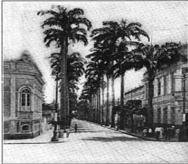
Para Tramways—Completed Track in Paved Street
