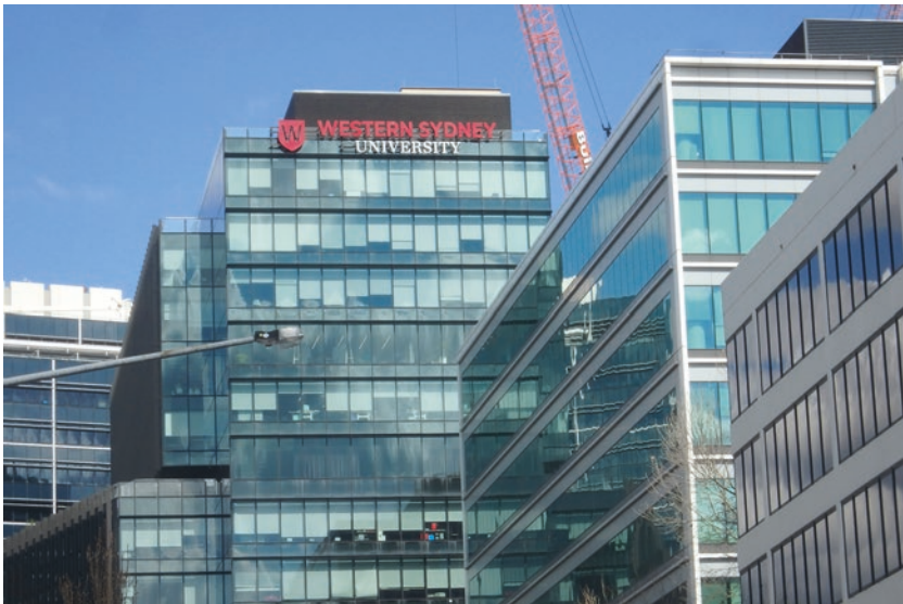
Fig. 6.7 Western Sydney University in Parramatta CBD
