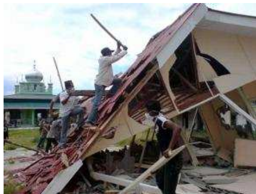
Figure 5.4: Asbestos-ridden houses torn down by their beneficiaries in Deah Raya village (courtesy of Komite Percepatan Pembangunan Perumahan dan Permukiman Desa)
