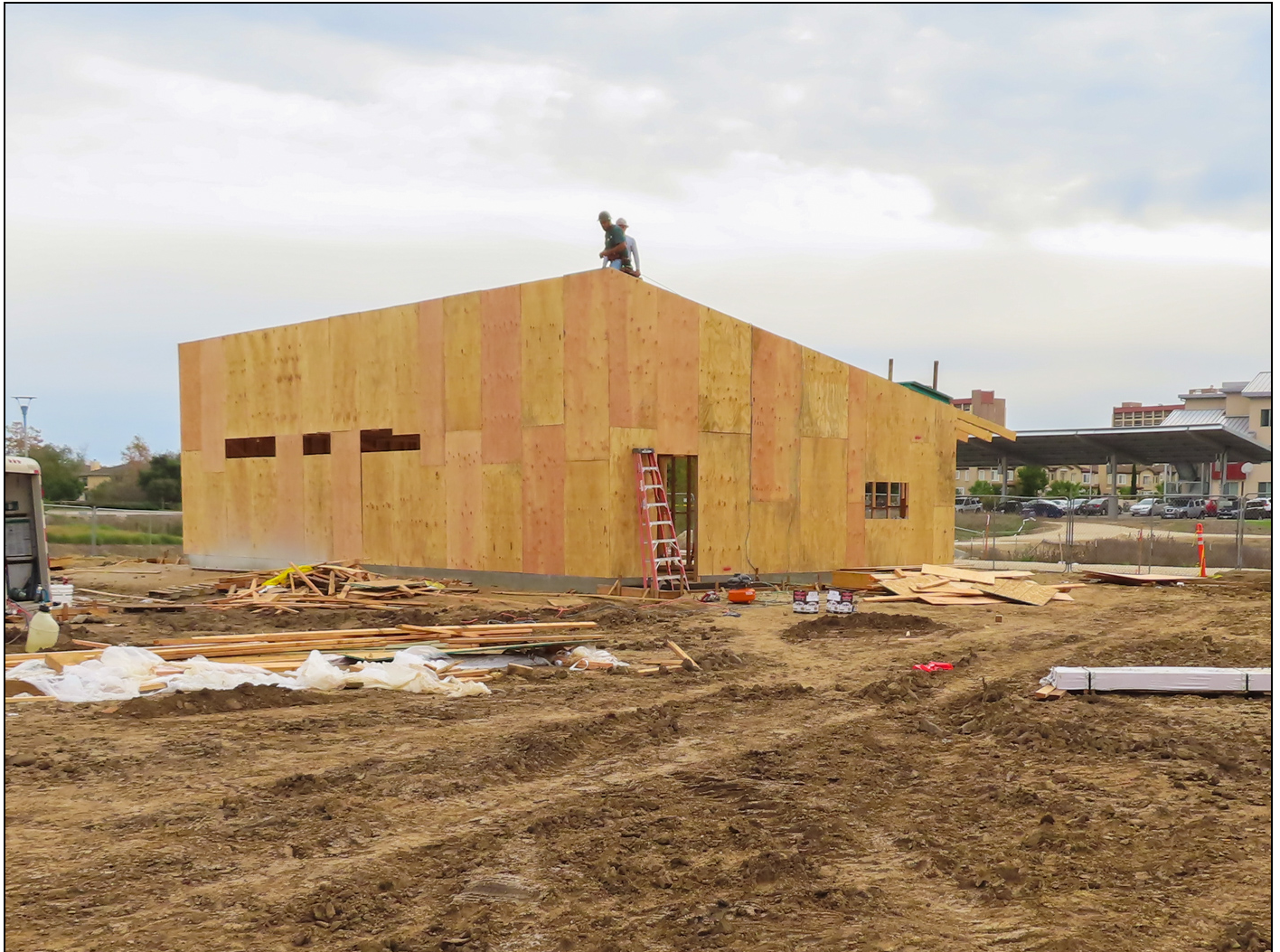
Construction of the NCOS 'Gator Barn'.
