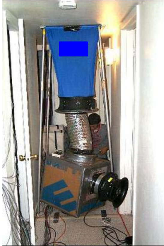
Figure 24. Multiple fan-flowmeter return powered flow hood
