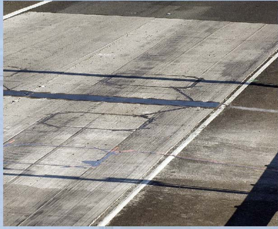
Figure 2 Cordelia Prototype VWS In-Ground Equipment
