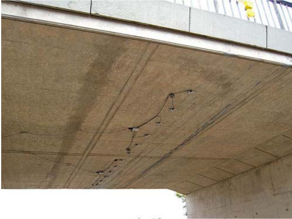
Figure 4 Strain Transducer to Underside of Bridge Structure
