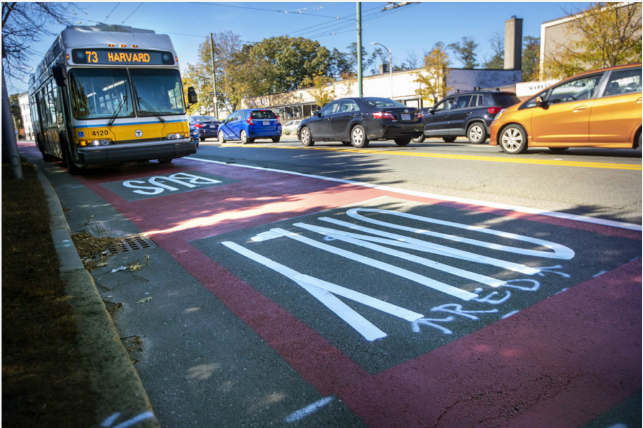
Cambridge/Watertown’s Mt. Auburn Street pilot TTL made their painted lane application temporary; the red paint is expected to disappear within months. Photo: Jesse Costa/WBUR
