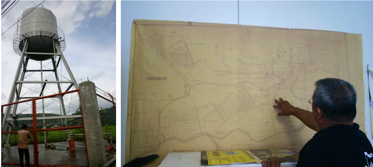
Figure 3.3. Pre-privatization micro-networks. Existing rural and peri-urban micro-networks tend to use their own groundwater sources to distribute water. To the left, a deep well and tank belonging to one cooperative. To the right, the chairman of another cooperative shows us a map of his service area. Photos by author.
