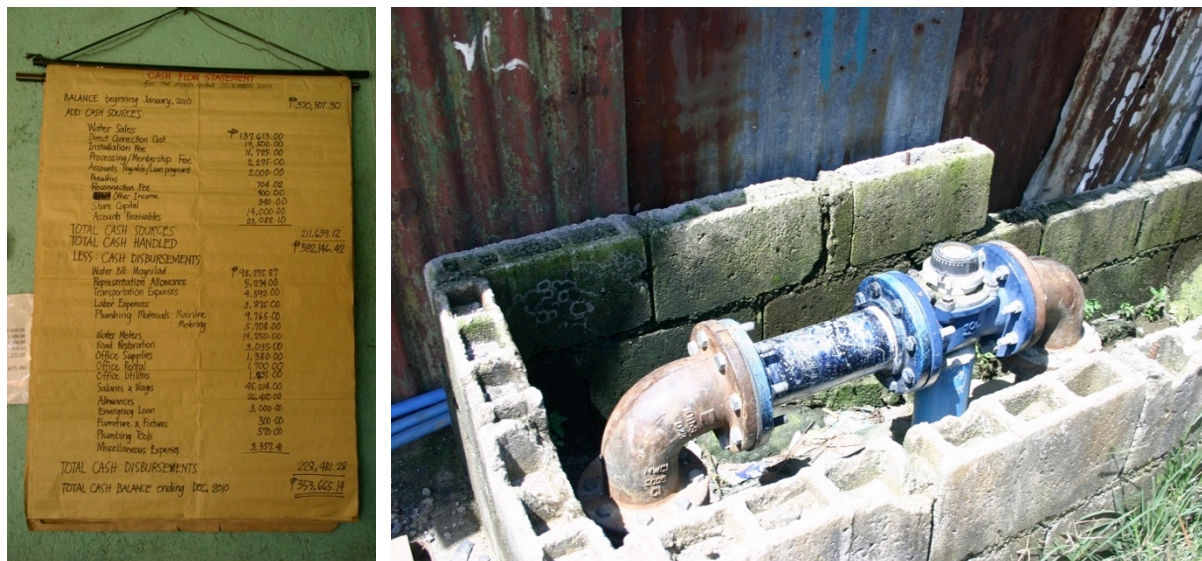
Figure 5.2. Micro-networks shift responsibilities from the concessionaires to CBOs. At left, micro-network operators maintain monthly budgets that must allow for full cost recovery. At right, bulk meters signal the end of the concessionaires’ territory and the beginning of the micro-networks’ infrastructure. Photos by author.
