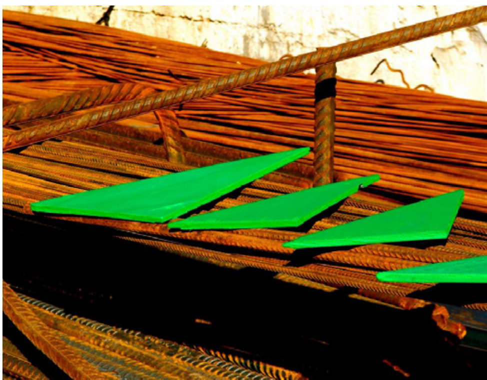
[Image 5] Study of Colors and Textures on the worksite. Mestres da Obra , 2013
