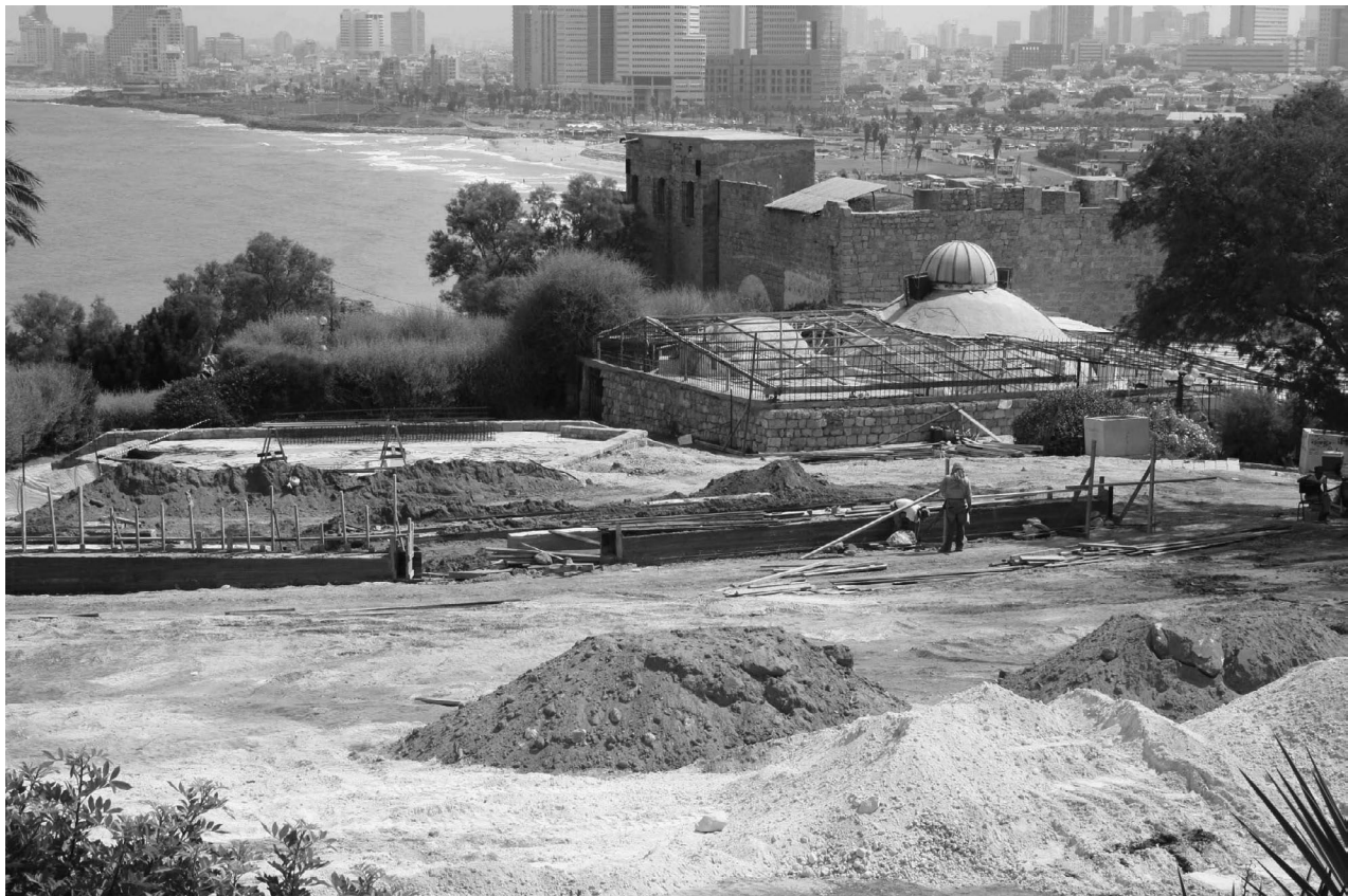
Figure 4.10. Renovation of the outdoor amphitheater in 2007.
