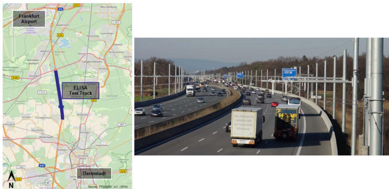
Figure 11. The ELISA pilot project in Germany. (Left) Map showing the location of the ELISA test track between Frankfurt Airport and Darmstadt, and (right) picture of the implemented catenary system.
