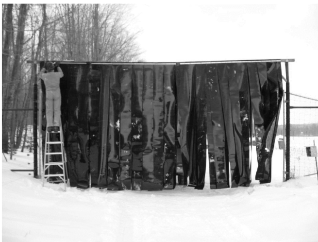
Figure 1. Installing the PVC curtain at a treatment site in Michigan, 2009.
