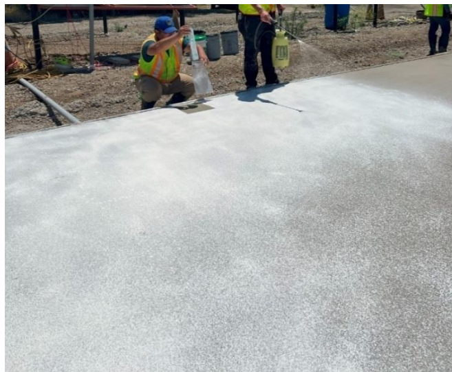
Figure 3.10: Curing compound application on portland limestone cement concrete (PLCC).
