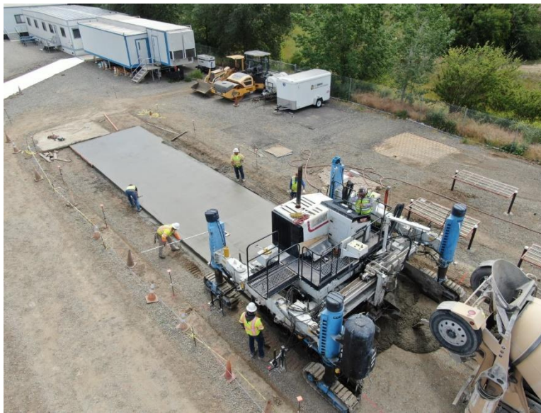
Figure 3.1: Lean concrete base (LCB) construction.
