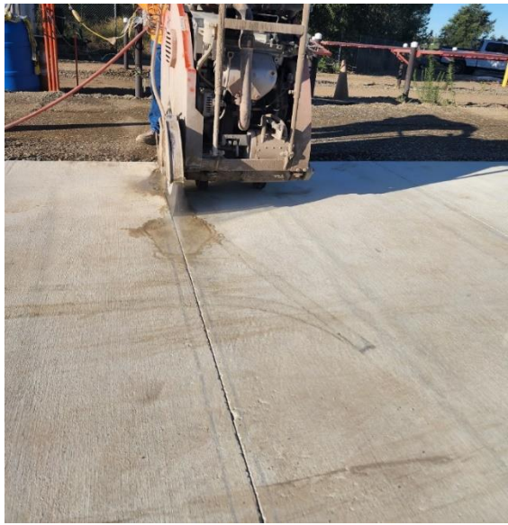
Figure 3.11: Full-depth cutting of transverse joints on portland limestone cement concrete (PLCC).
