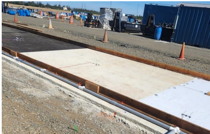
Figure 3.5: Section with curing compound bond breaker before portland limestone cement concrete (PLCC) paving.
