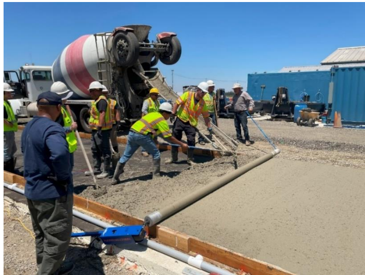
Figure 3.9: Portland limestone cement concrete (PLCC) construction.
