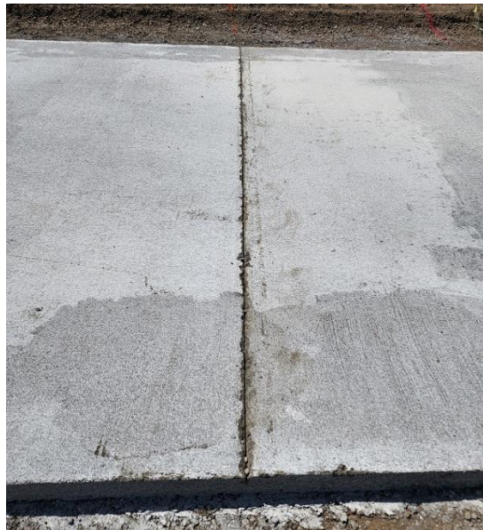
Figure 3.3: Lean concrete base (LCB) partial depth saw-cut.
