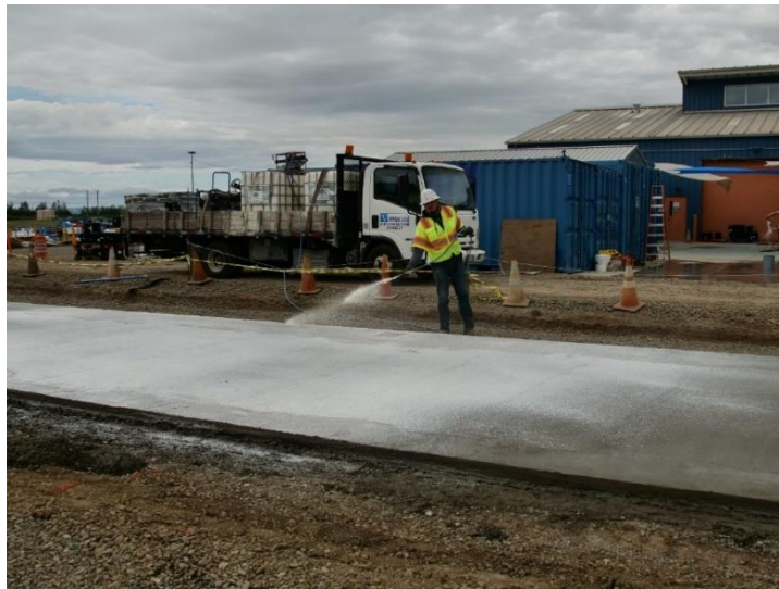
Figure 3.2: Curing compound application on lean concrete base (LCB).
