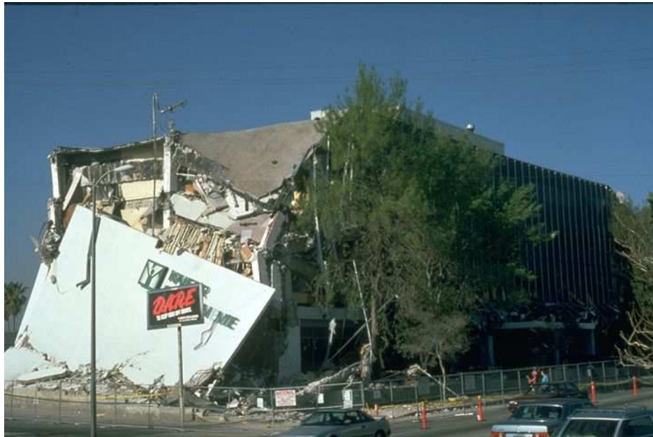
Figure 1.1: Partial collapse of Kaiser Permanente office building after 1994 Northridge earthquake.
