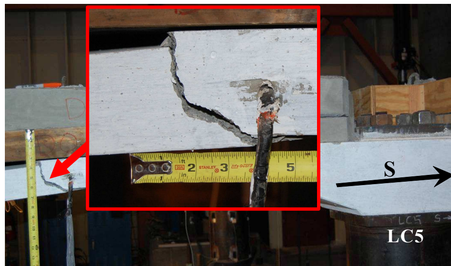
Figure 3.21: Localized failure near LC5 during test at slab-slab corner of specimen 1.
