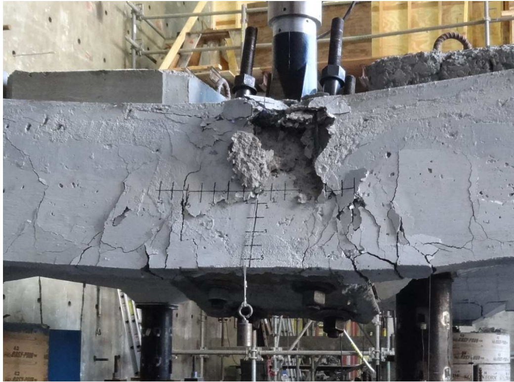
Figure 3.43: Local failure at beam edge push location creating large torsion in the beam.
