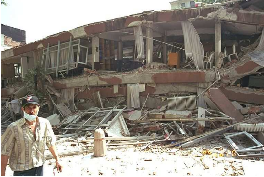
Figure 1.2: Collapse of a concrete structure during the 1999 Izmit earthquake, Turkey (photo courtesy: Halil Sezen).
