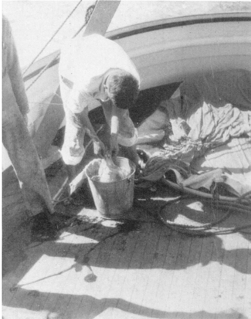
FIG. 23. Before the net is hauled to the deck, it is given a good swashing to drive the clinging material into the silk tip. It is then hauled aboard and the silk bag inserted in a pail of water, where the entire contents are washed into the glass jar inserted at the tip. Photograph by Donald H. Fry, Jr., 1931
