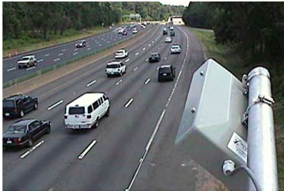
Figure 6 - Multi-lane highway monitoring using SAS-1
