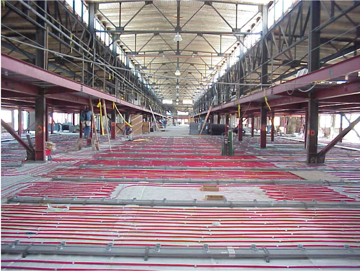
Figure 7.4 Radiant system (WSP Flack and Kurtz 2007).
