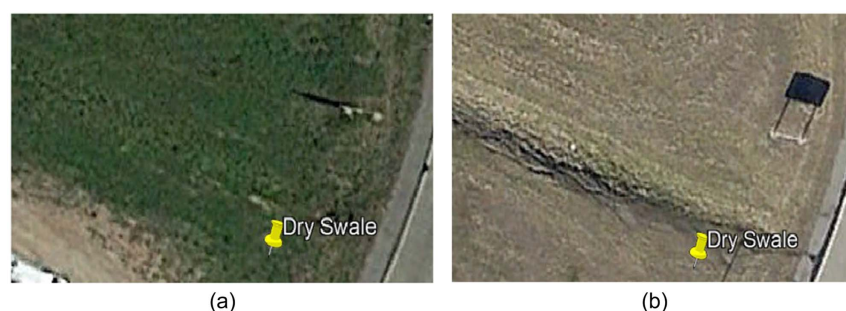
Fig. 1. Satellite image of the same grass swale in April of (a) 2014; and (b) 2013. Dry swales need a pretreatment area (e.g., grassed filter strips) to catch coarse sediment and prevent clogging of the engineered soil mix. Fig. 1(b) shows signs of degradation of the filter strip, pointing to the degradation of BMP efficacy. (Images © Google Earth Pro.)
