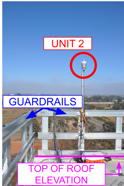
Figure 6: Unit 2 installed above the roof level of the CFS10 specimen during seismic test.
