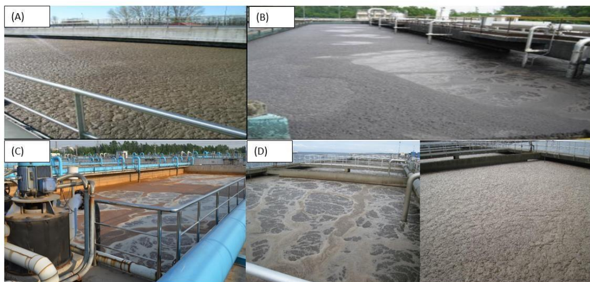
Figure 1.3: Impact of ozone on controlling foam formation: A) foam formation in waste water treatment; B) reduced foam formation by Ozonation (Ried et al. 2014); and C,D) Ozone treatment of wastewater. Modified online images [A, B, C, D]. Available from: https://www.semanticscholar.org/paper/Ozone-to-Control-Bulking-and-Foaming-in-Municipal-Ried-Wang/8023d02b3ef143cb5eb072cac029ce17b8945df4/figure/2 ; https://ozonesolutions.com/wastewater ; https://www.semanticscholar.org/paper/Application-of-ozone-in-wastewater-treatment-%3A-For-Nilsson/9947e5257ee1a79f5381b7899446a6d58e9d7ff1#extracted . [Accessed 3 December, 2023].
