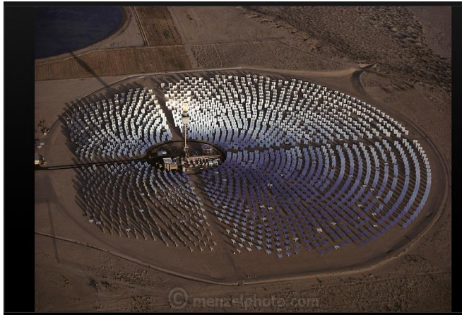
Figure 3 shows a large concentrated solar thermal energy collection setup. Three of these setups currently reside in the California Mojave Desert [4].
