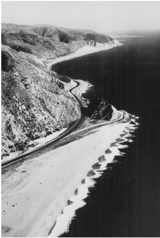
Fig. 5. Effect of headlands on the accretion of beach sand at Point Mugu, California. The point forms a natural obstruction that interrupts the longshore transport of sand, causing accretion and a wide beach to form (foreground). The regularly spaced scallops are swash cusps on the beach face. (Department of Engineering, University of California, Berkeley)
