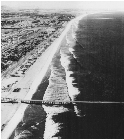
Fig. 1. Longshore currents, generated when waves approach the beach at an angle. At Oceanside, California, the longshore current is flowing toward the observer. (Department of Engineering, University of California, Berkeley)
