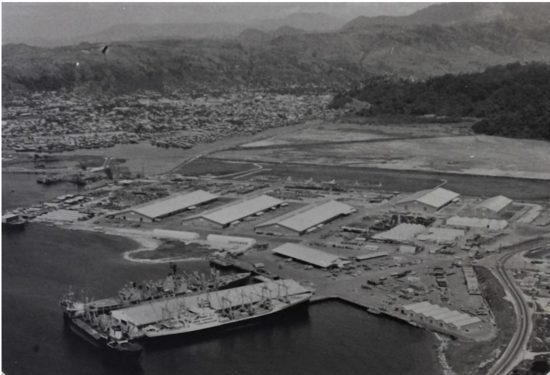
Figure 2-3 Naval Supply Depot Storage/Terminal Complex. Background Olongapo City, 1969. 91
