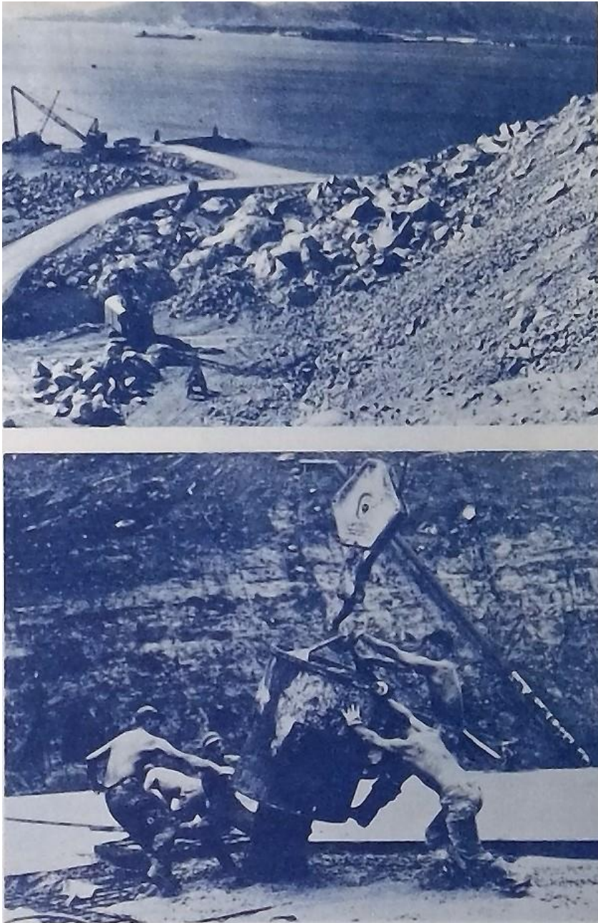
Figure 2-6: Materials and sounds: U.S. Naval engineers build Cubi Point, circa 1950s. 121
