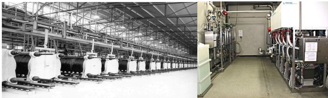
Figure 3: 135 MW KOH electrolyzer plant on left and 1 MW PEM system on right
