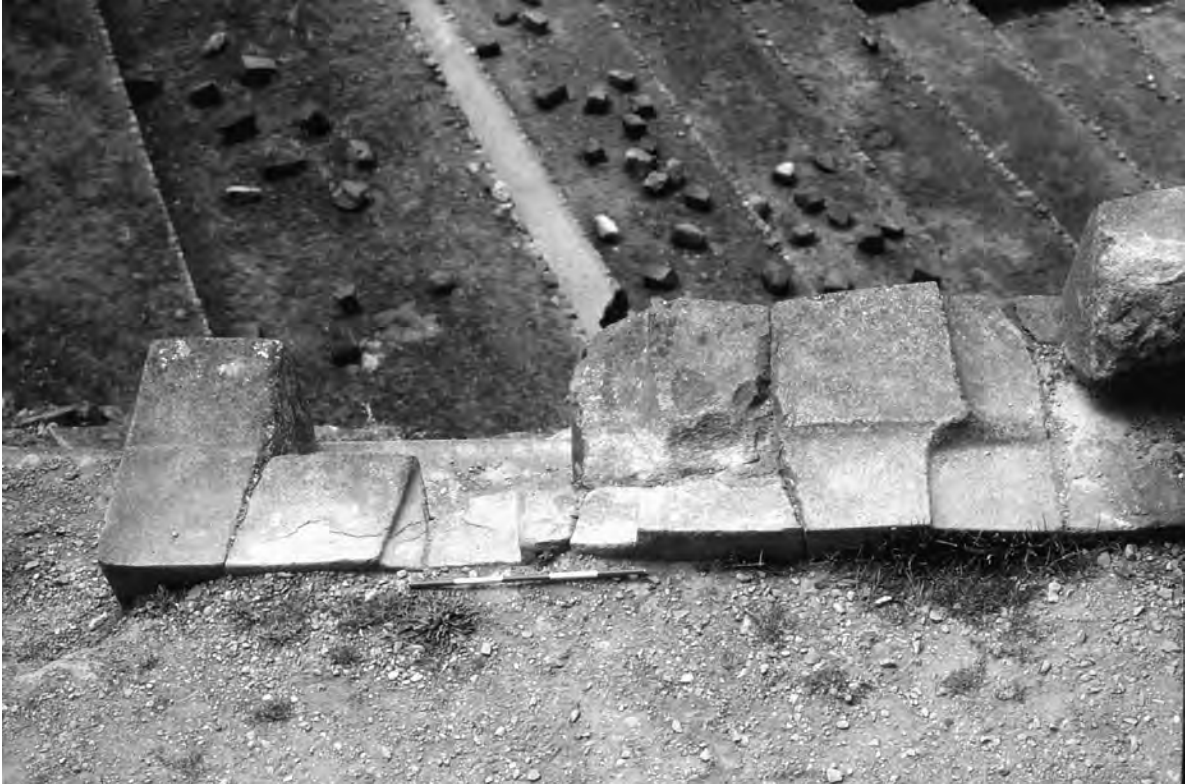
Figure 2.72. Imprints left by removed stones in Inca masonry.
