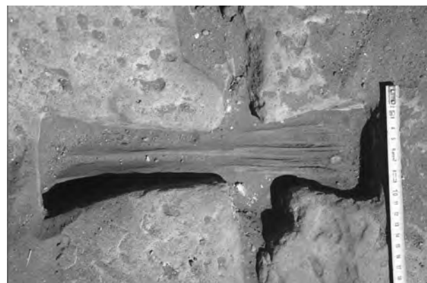
Figure 6.23. Wooden dovetail cramp at the temple of Khnum, Aswan.
