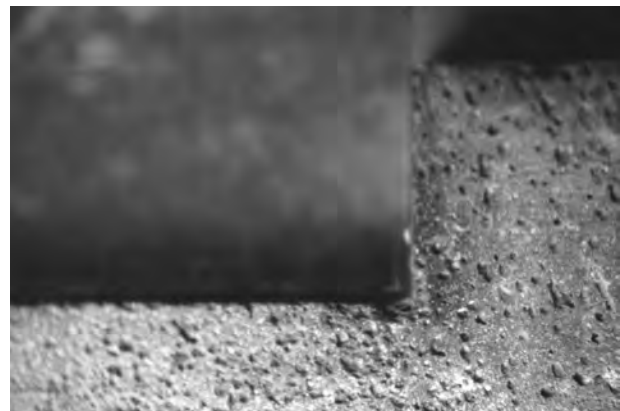
Figure 5.14. Close-up of finished corner in the motif, revealing the precision obtained in the form of a perfect right angle. Note also the damaged surface of the interior angle where Nair learned how fragile this area is, and hence, the need to preserve this area until the very final stages in the carving.
