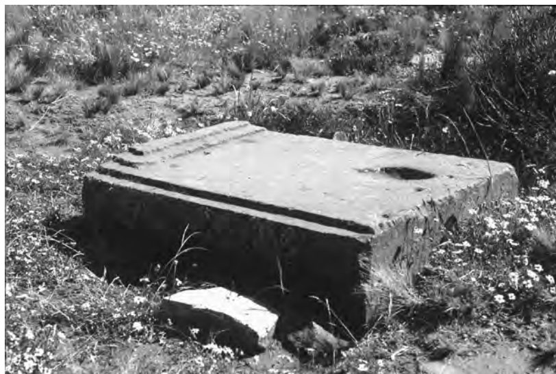
Figure 3.86. Possible jamb stone of Akapana Gate.
