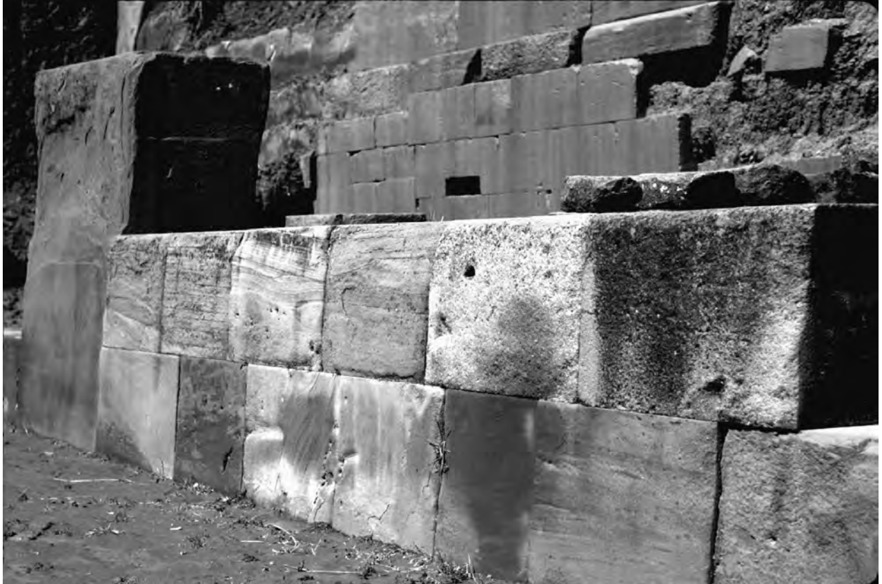
Figure 2.10. Second wall of Akapana's east side.
