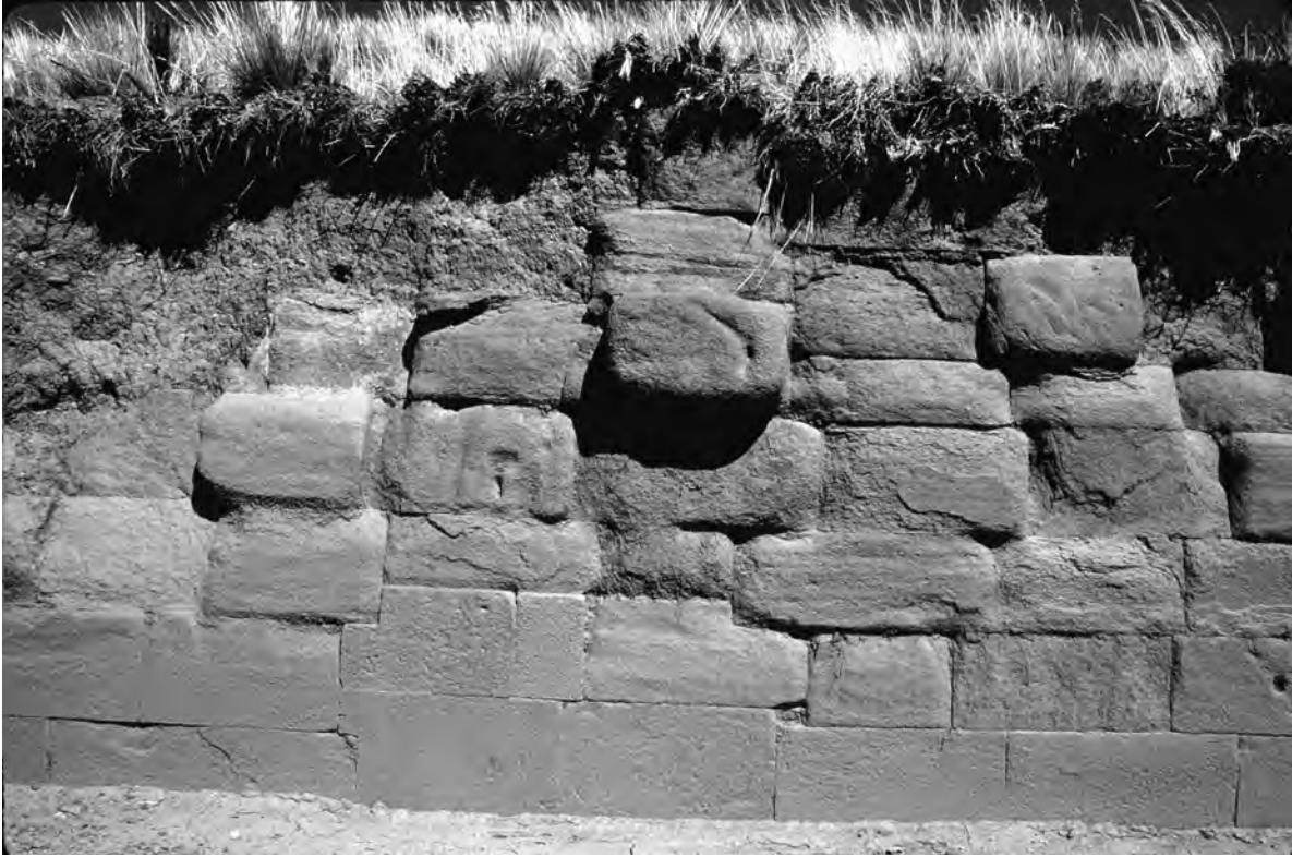
Figure 2.25. Third wall masonry detail and tenon, Akapana's north side.
