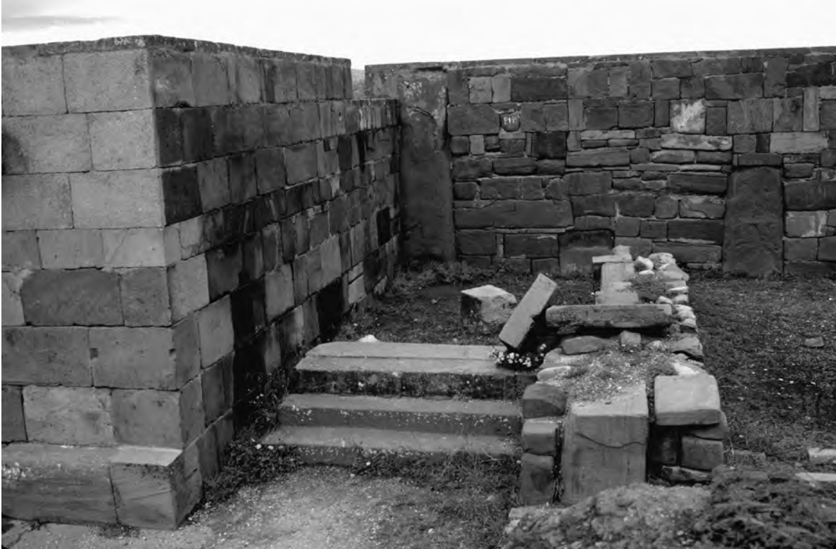
Figure 2.35. Stairs on south side of Balcony Wall.
