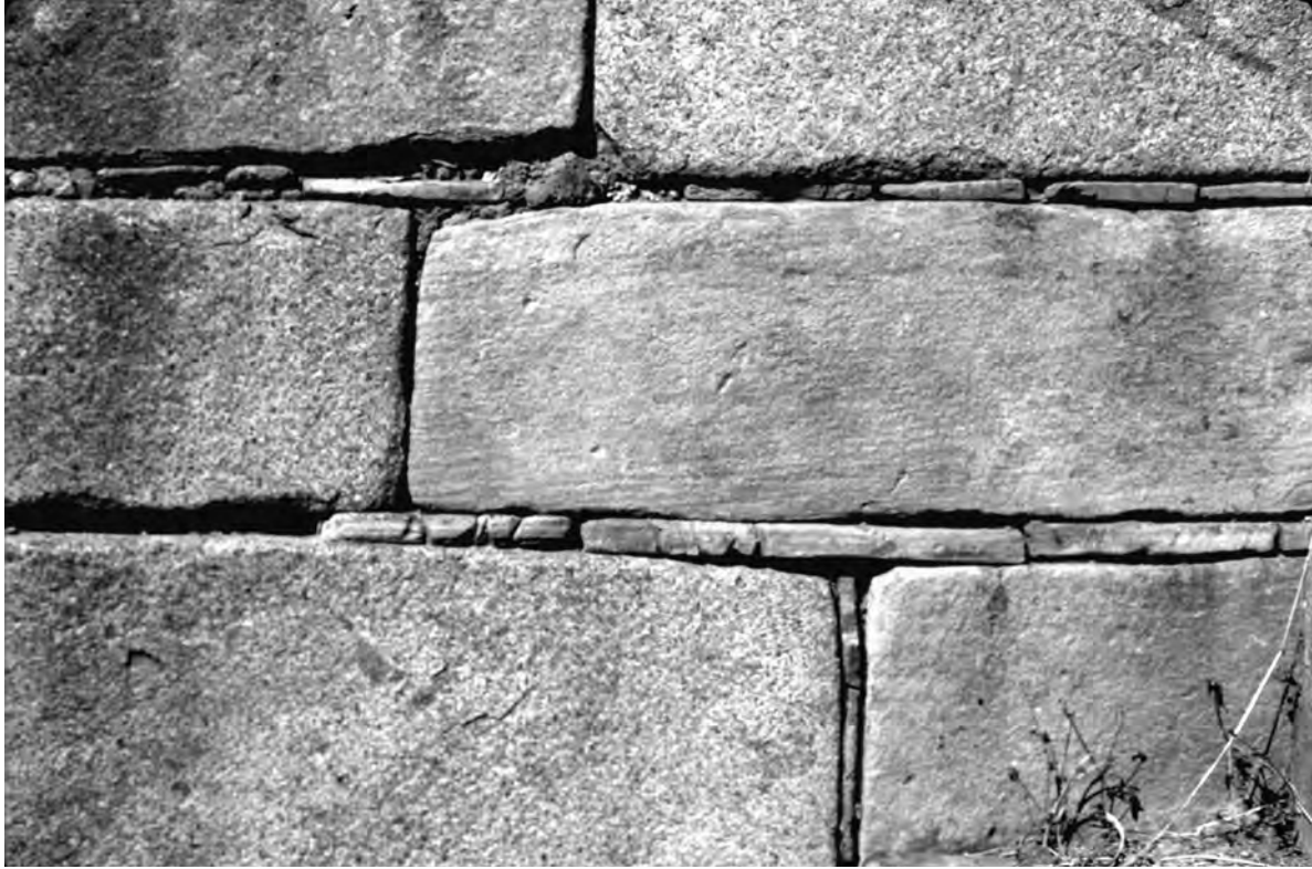
Figure 2.70. Chinked cut-stone masonry at Chavín de Huántar.
