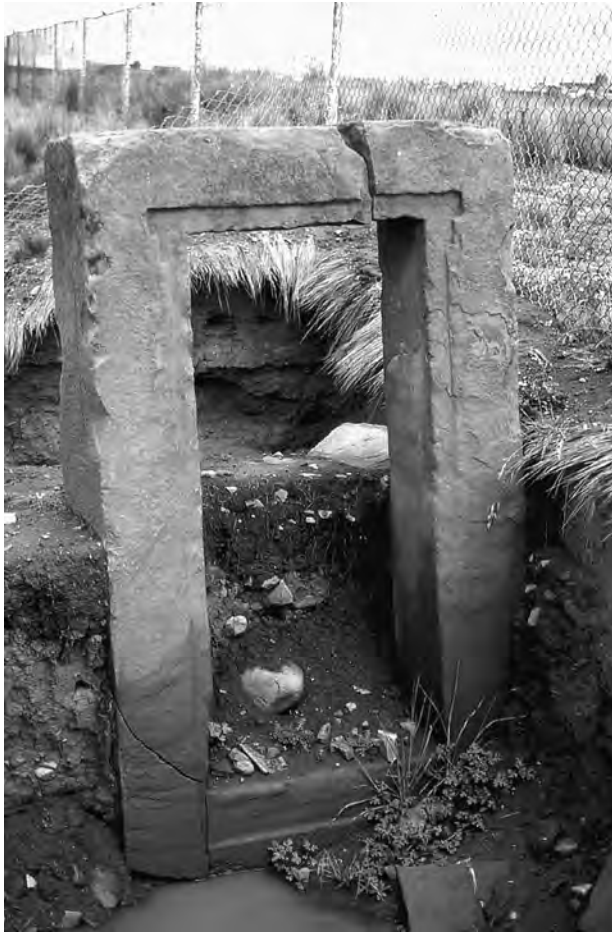
Figure 3.90. Sandstone Gateway, view of east (or front) side.
