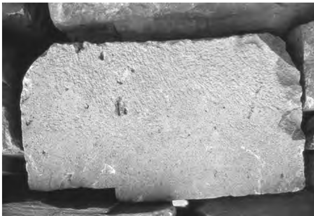
Figure 5.27. Stone Type 4.3 in the Akapana, showing chisel marks.
