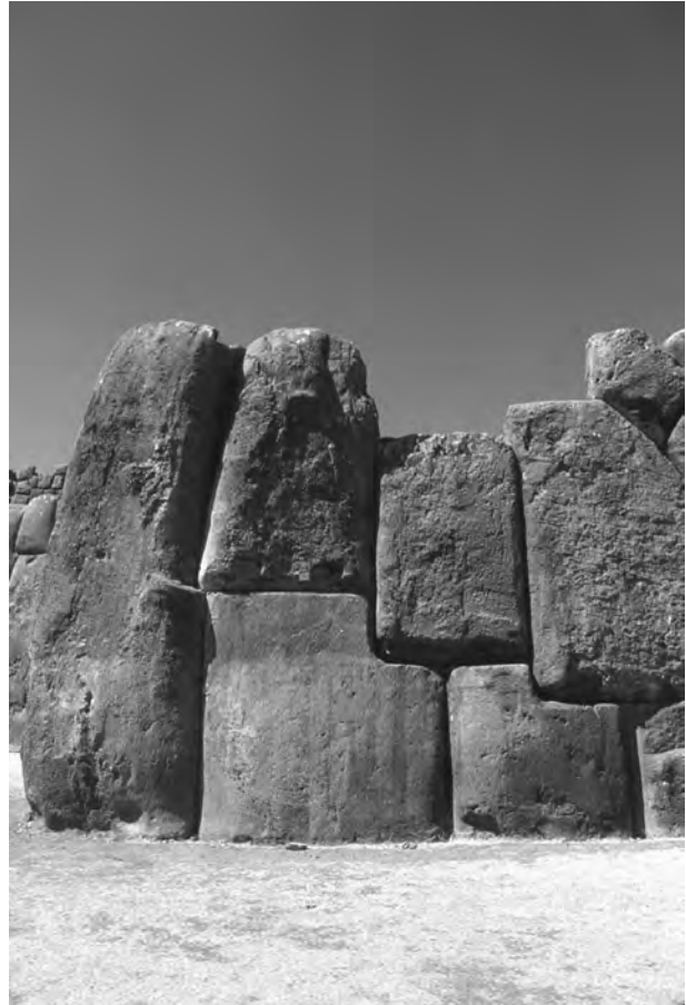
Figure C.2. L-shaped joints at Saqsawaman.
