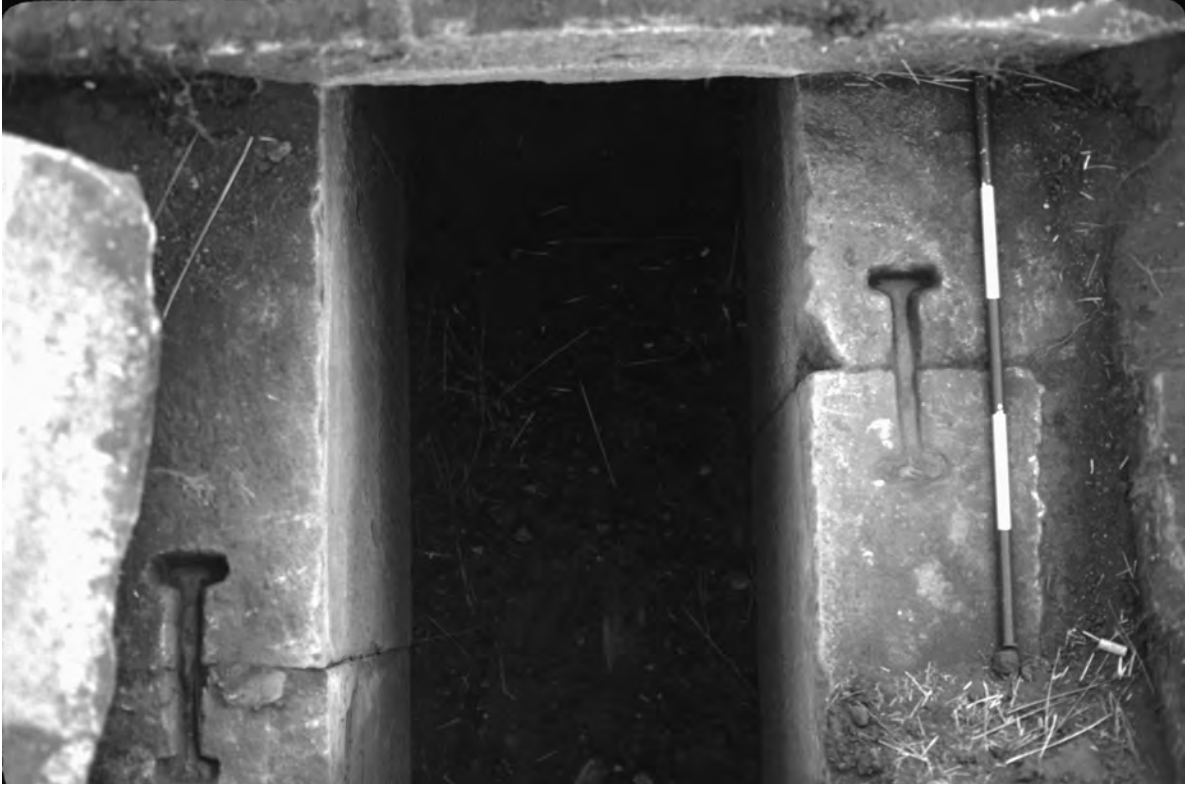
Figure 2.64. Cramps in situ in canal on Pumapunku's south side.
