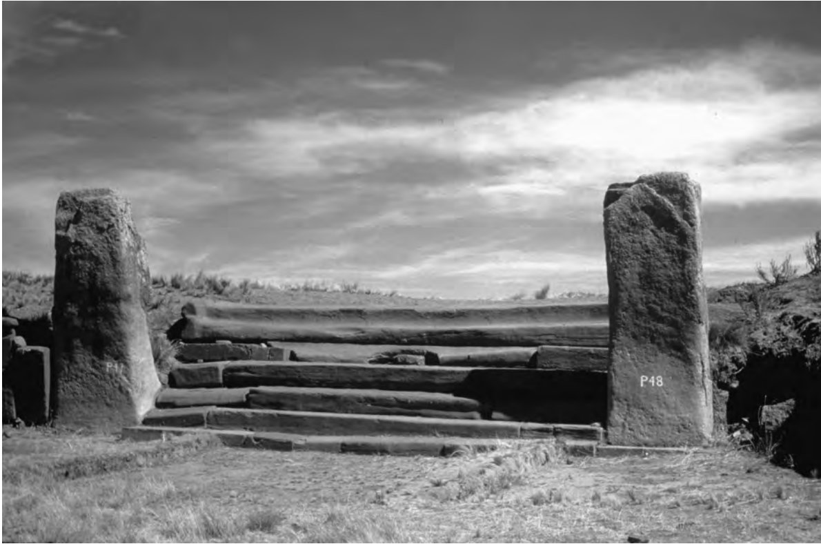
Figure 2.32. Stairway to Kalasasaya east before reconstruction (photo anonymous).
