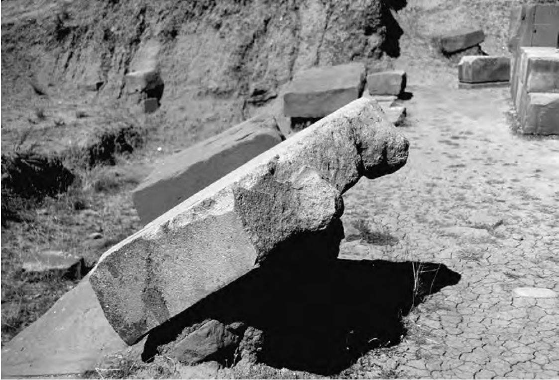
Figure 6.13. Protuberances or bosses to handle stones.
