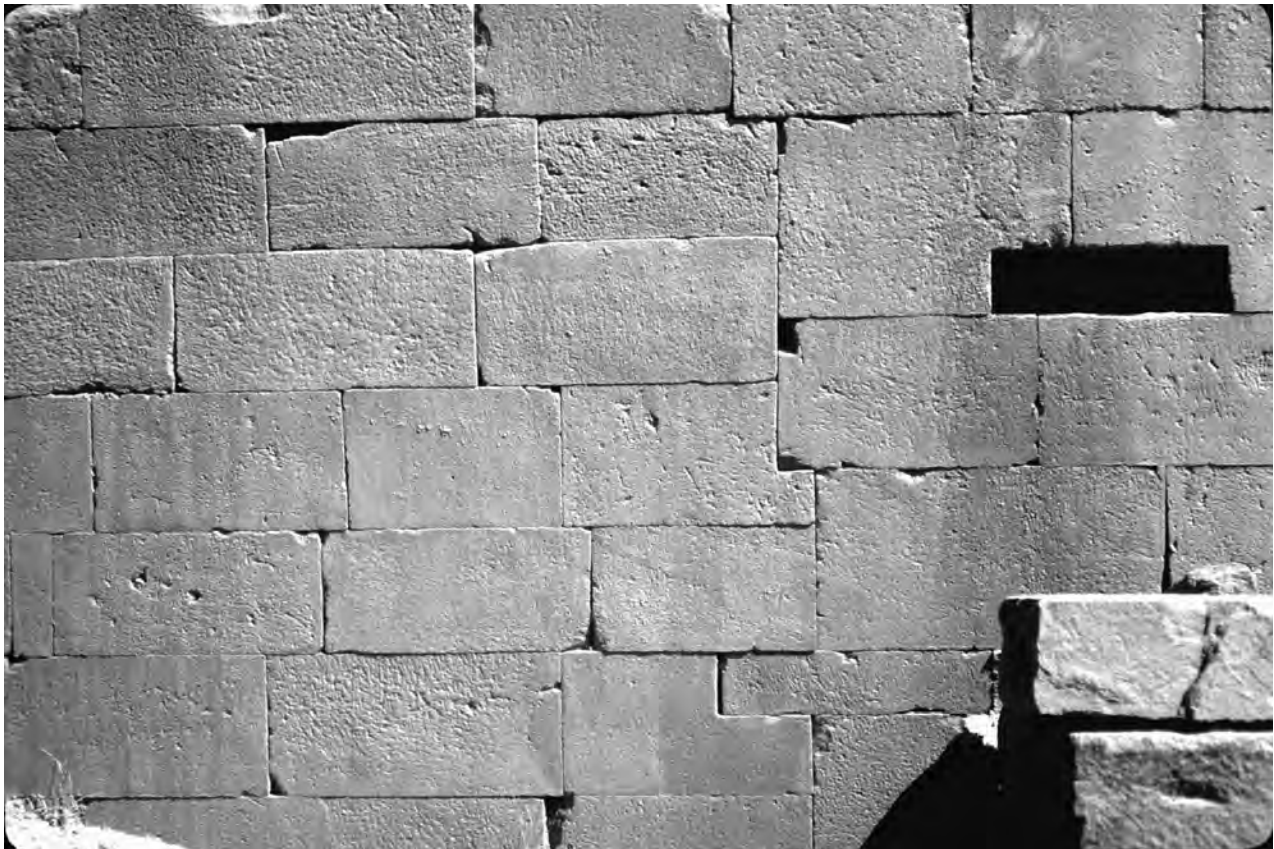
Figure 2.12. Quasi-coursed masonry of third wall of Akapana's east side.
