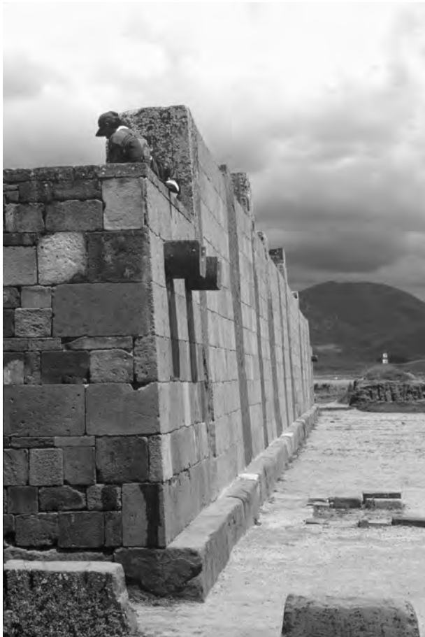
Figure 6.19. Sandstone blocks as foundation under the Balcony Wall.
