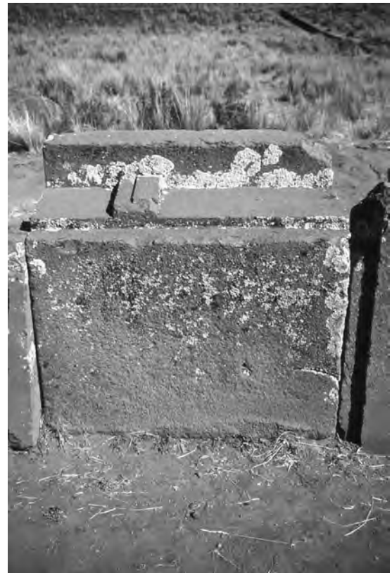
Figure 3.23. Jamb stone with step molding.
