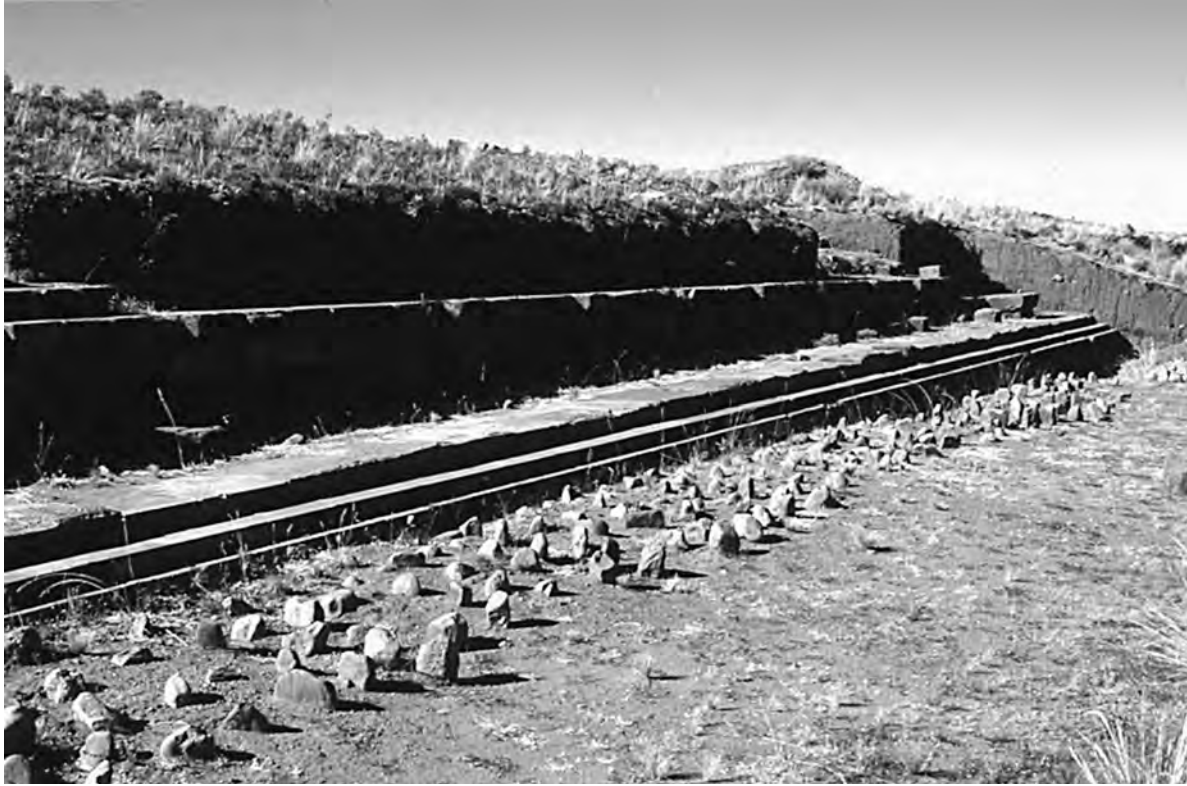
Figure 2.46. Stereobate and second terrace wall on Pumapunku's south side with soil nails at the base.
