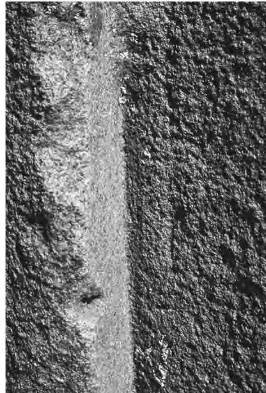
Figure 5.20. Note that the corner is made ever tighter toward the bottom. The round tool marks are replaced by sloping lines. These chisel marks show the transition to an ever smaller and more easily controlled tool head. Note also that the plane to the left of the corner is smooth (pock marks of a small hammer tool), while the plane to the right of the corner is rough (pock marks of large- and medium-sized hammer tool).
