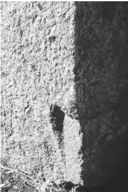
Figure 5.16. Note how a flattened, planar surface is transferred to an adjacent face of a stone block.
