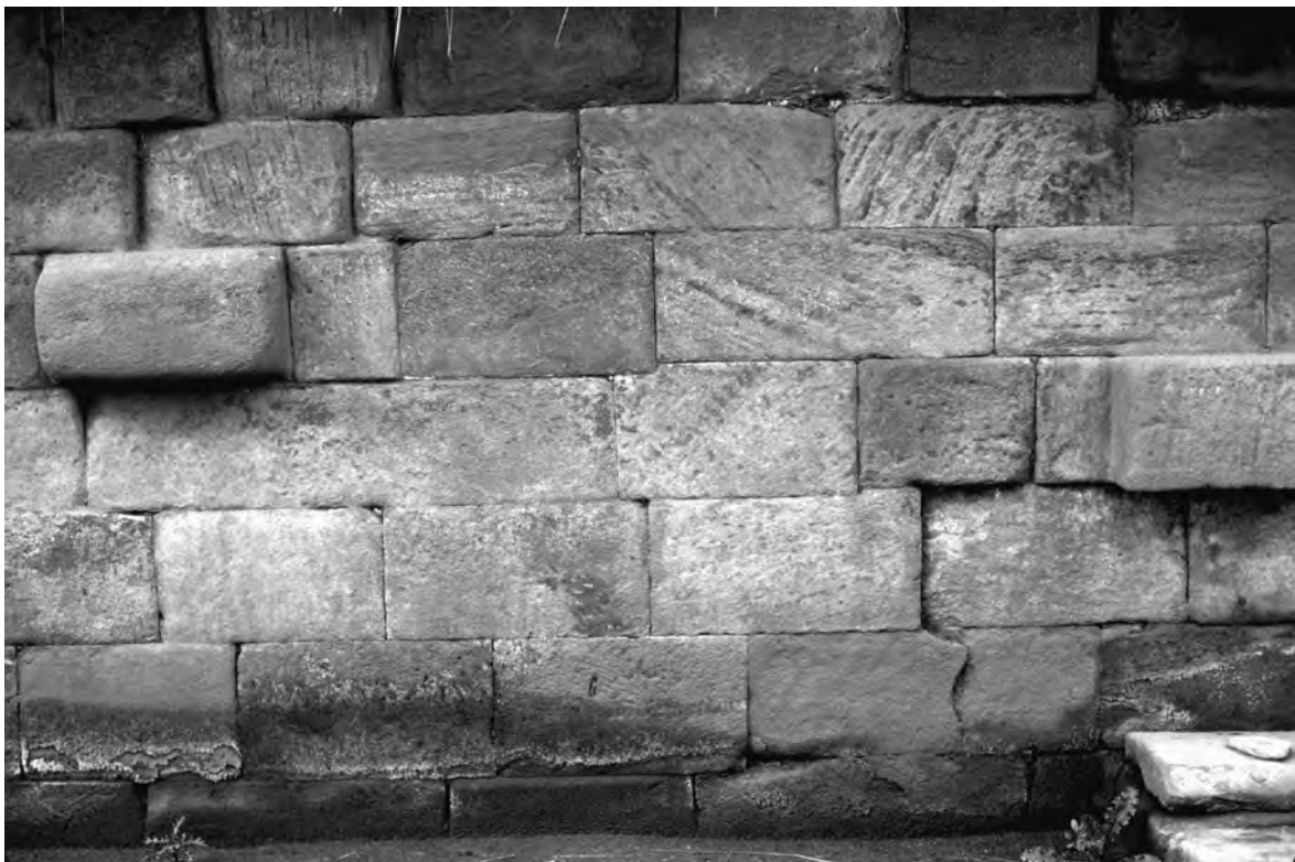
Figure 2.18. Quasi-coursed masonry of second wall on Akapana's south side.
