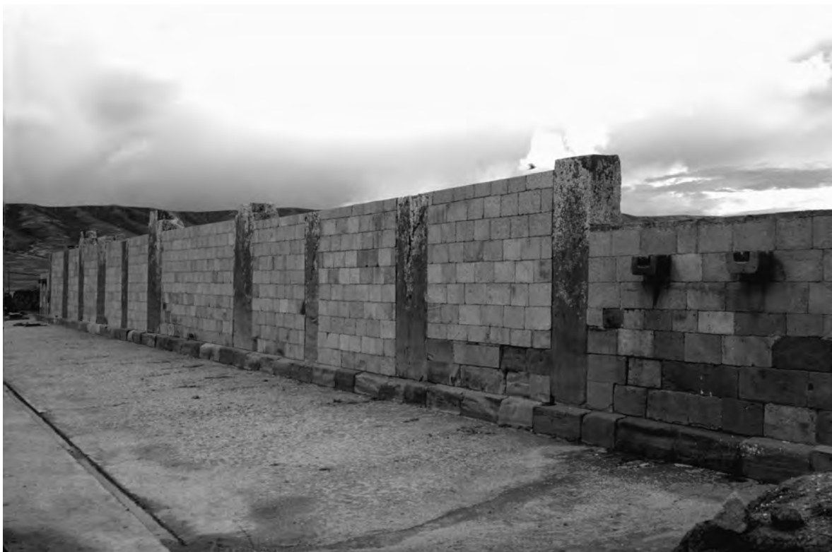
Figure 2.38. Balcony Wall (from southwest).
