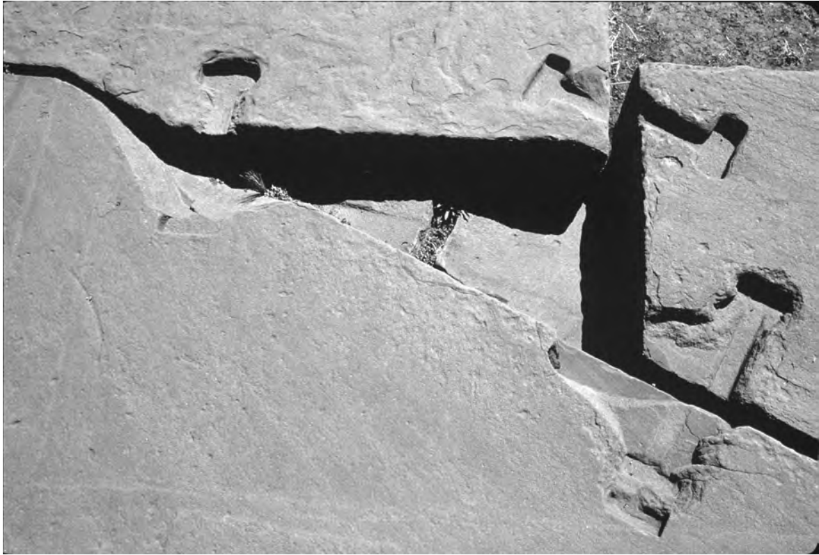
Figure 6.25. Cramp sockets on Platform III at Pumapunku.
