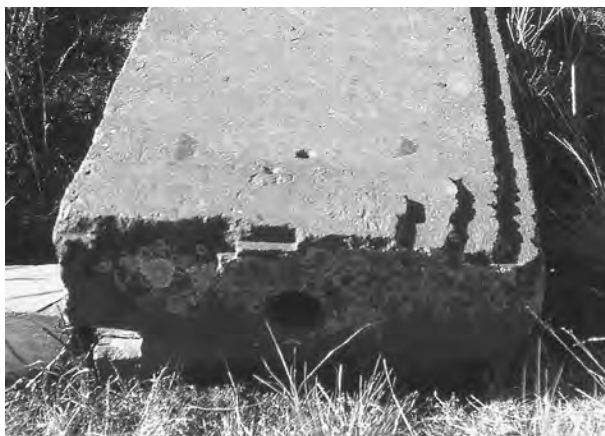
Figure 6.27. Recessed cone in jamb of the Akapana Gate.
