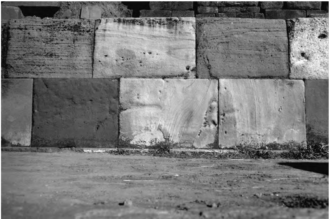
Figure 2.11. Opus quadratum of second wall.
