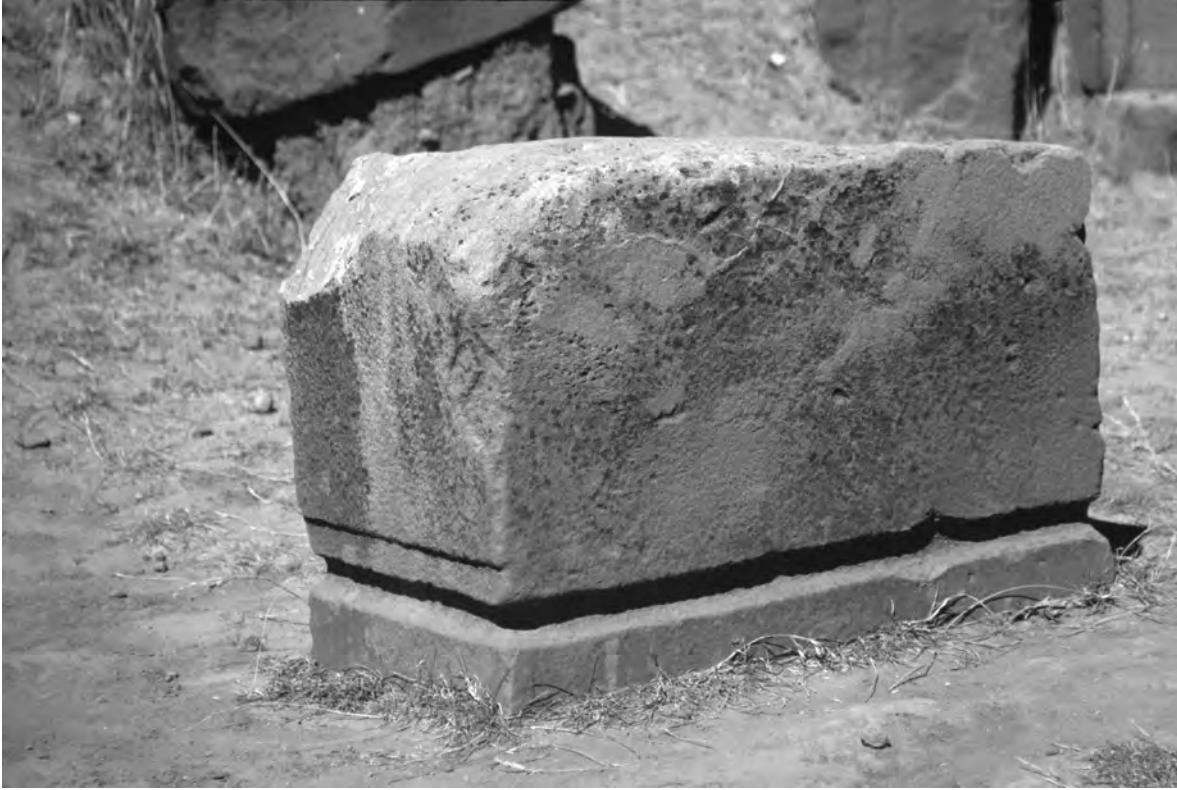
Figure 6.15. Rope chases.
