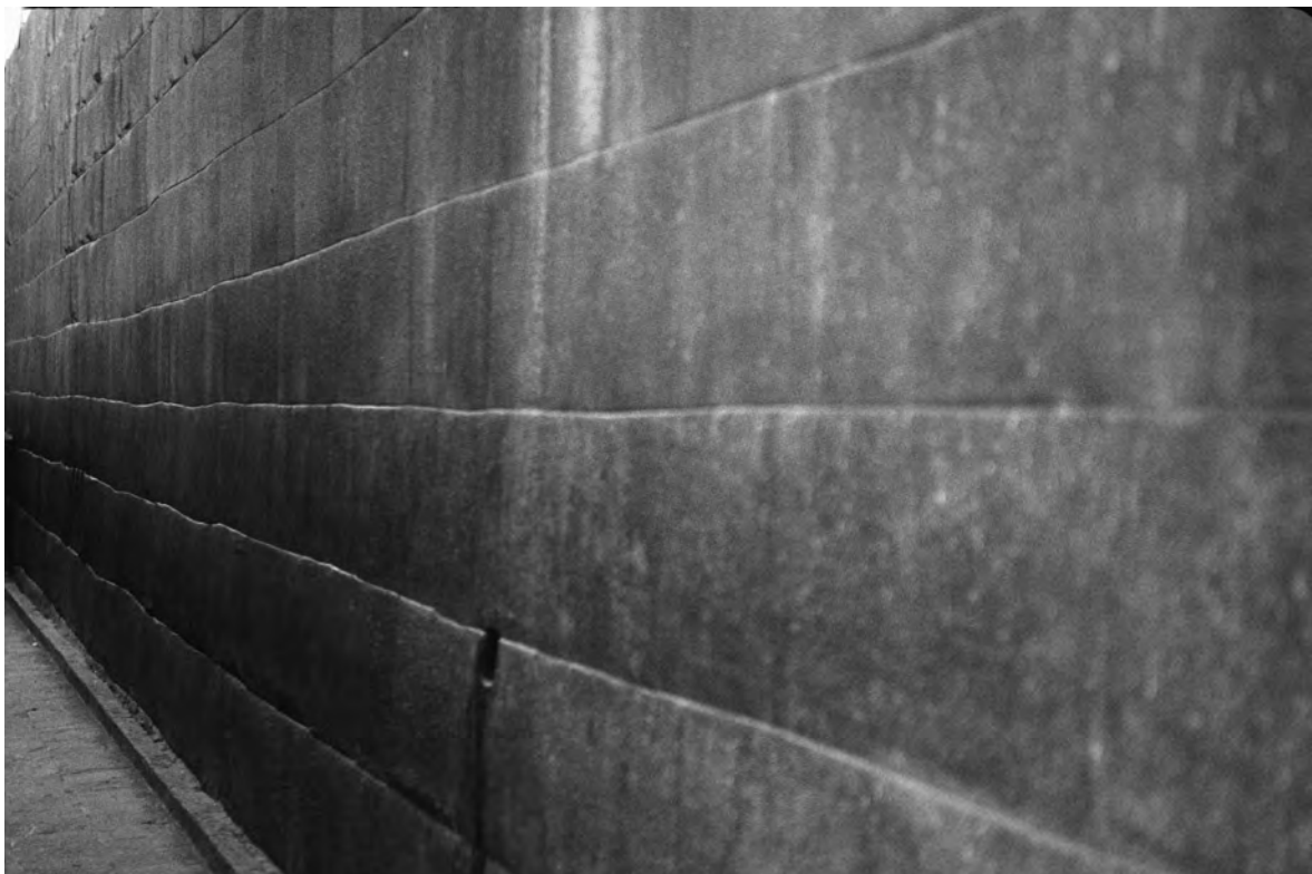
Figure 2.71. Wavy horizontal joints in Inca ashlar masonry.
