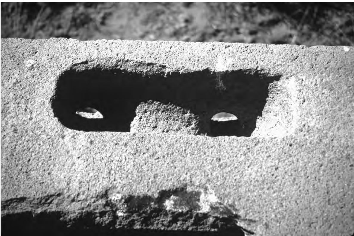
Figure 6.17. Hoisting grip.
