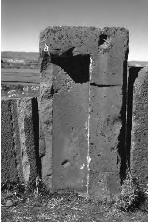
Figure 3.28. Lintel stone with recessed panel.
