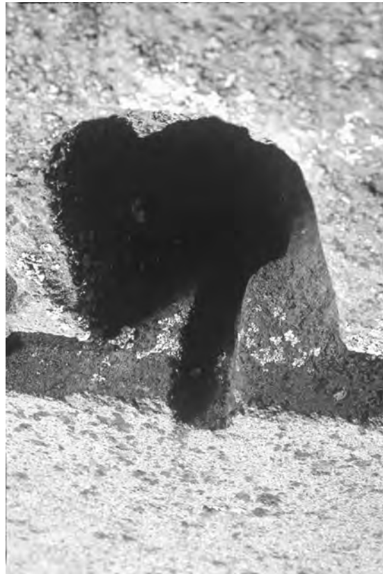
Figure 6.26. Recessed cramp socket.
