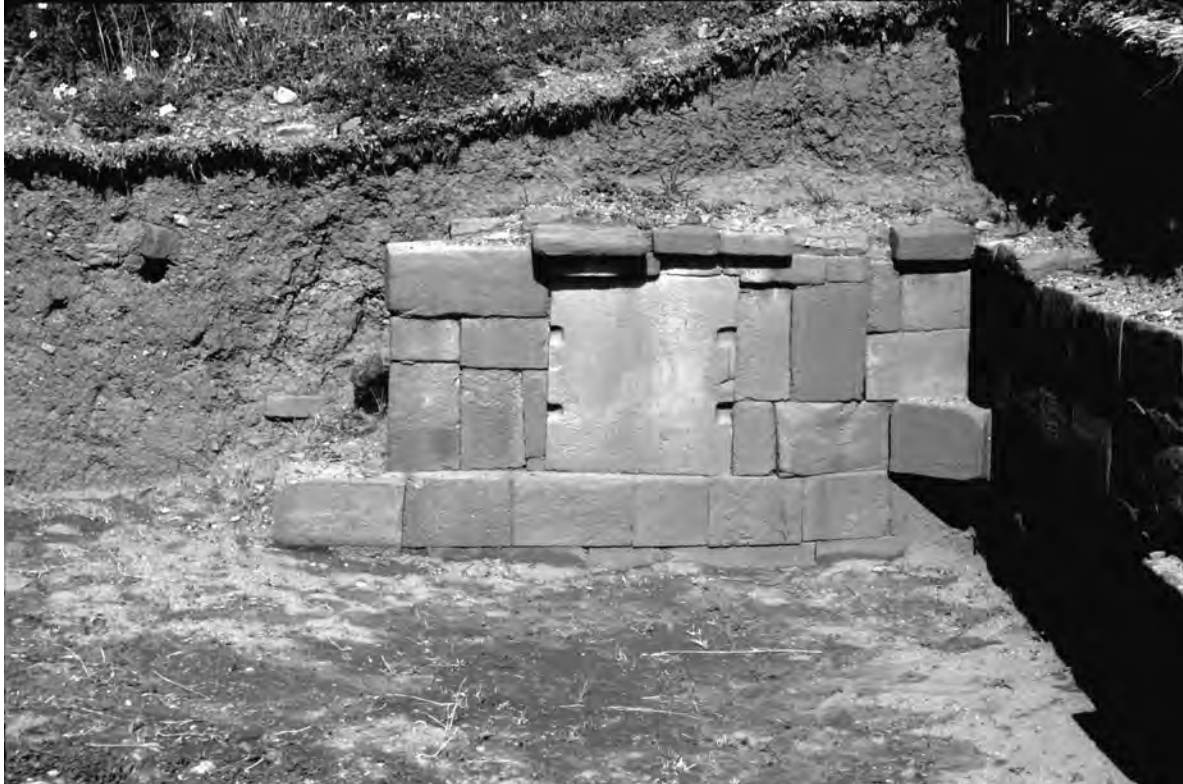
Figure 2.23. Third wall with reused stones and a stone set diagonally across the inside corner.
