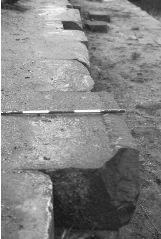
Figure 6.10. Residual bulges on second tier wall, suggesting in situ fitting.
