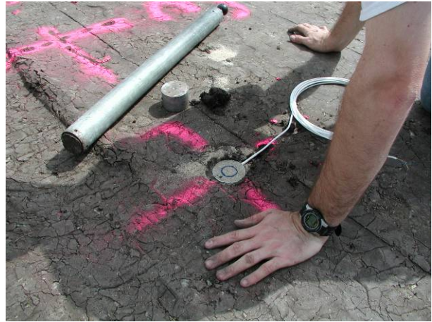
Figure 2.9: Installation of pressure cell
