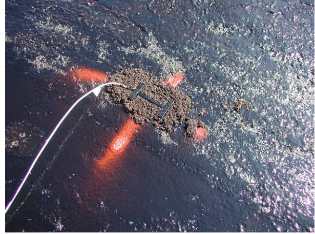
Figure 2.12: Installation of strain gauges
