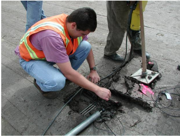
Figure 2.8: Installation of Time Domain Reflectometer
