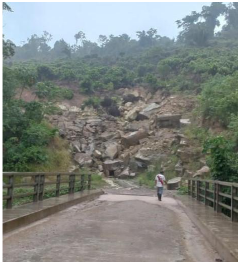
Figure 18. A Lucanyacu community member examines the aftermath of the landslide that covered the road to the Lucanayacu bridge. Photo by Maestro Orlando Chujandama.
