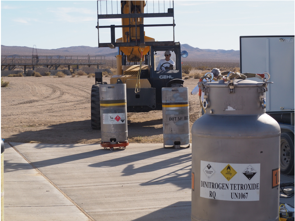
Figure A.6: Reach for positioning propellant drums near test stand for propellant load.
