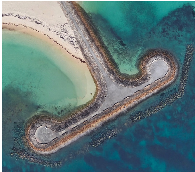
Close-up of Nishihara Kirakira Beach's groin-jetty structure with the most visible part in natural stone hiding tetrapods piled on a submerged breakwater offshore. Source: Google Maps.
