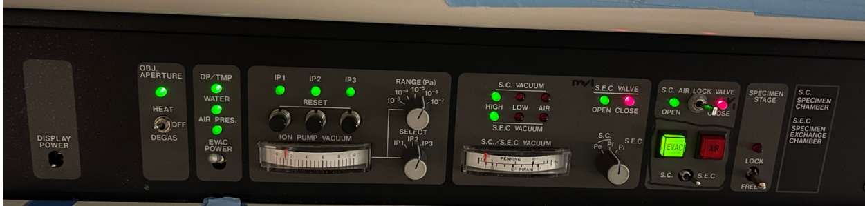
Figure 4. 1. Valve, switch and green light shows operational SEM conditions.
